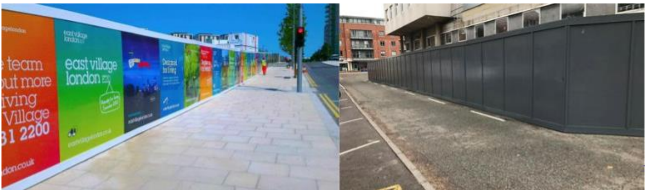
Figure 7 - Examples of hoarding
