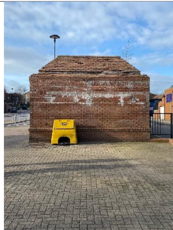
Photo 12 – Building B eastern aspect
