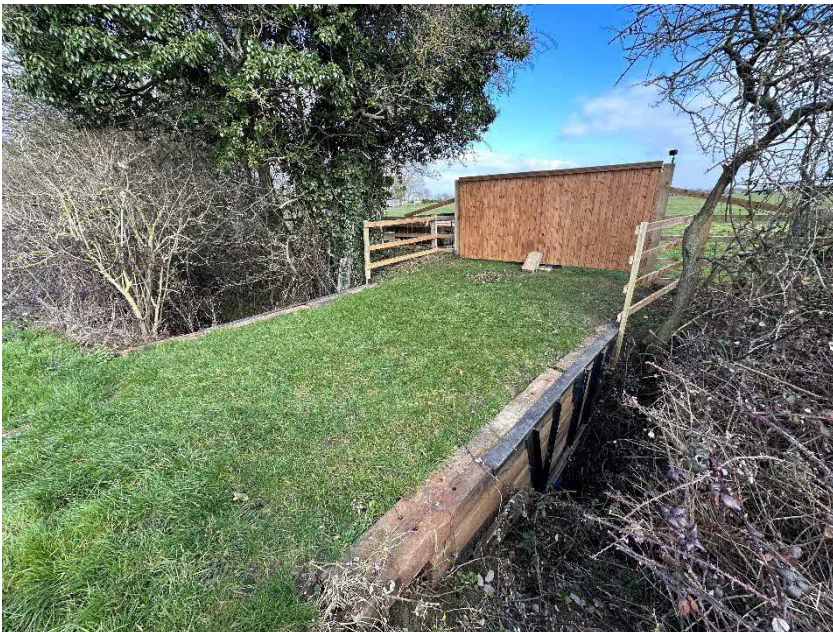
Access from the rear of the house over the existing culverted drainage ditch.
