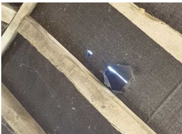
Photograph 9 and 10: Tears in the felt lining corresponding with gaps in the slate tiles above
