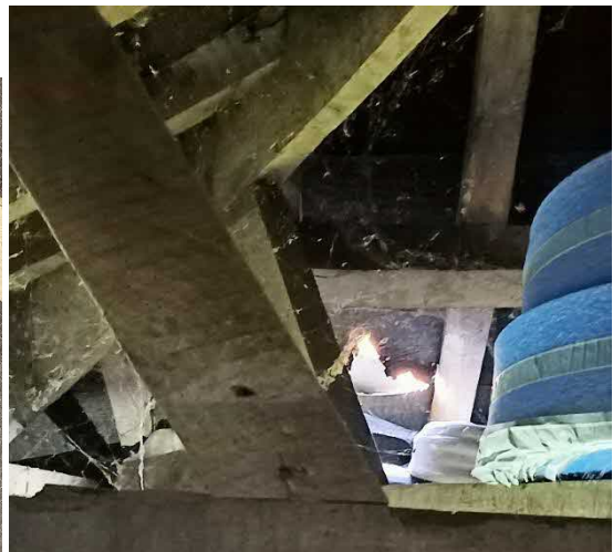
Photograph 9 and 10: Tears in the felt lining corresponding with gaps in the slate tiles above
