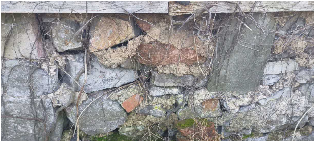
Photograph 6: The middle section of the northern stone wall, showing gaps within the mortar providing crevice roosting potential
