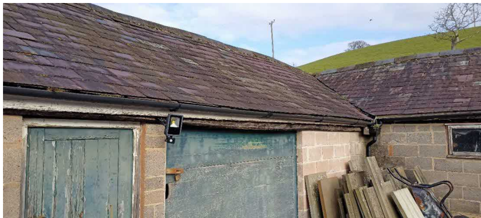
Photograph 2: Southern aspect of the outbuilding, showing one of the security lights
