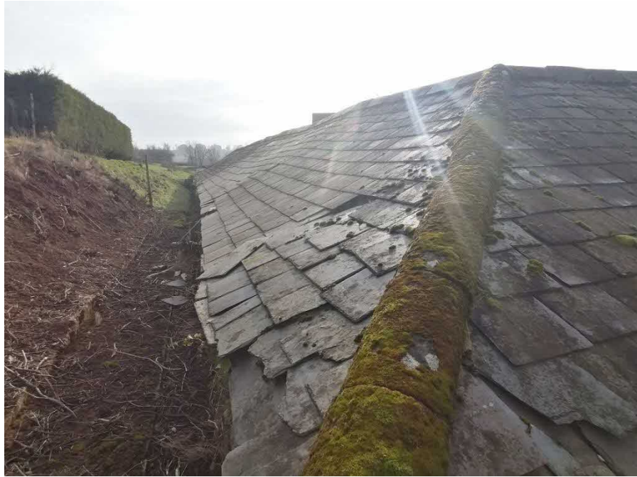
Photograph 4: North eastern corner of the outbuilding, highlighting multiple broken and lifted tiles along the eastern aspect and corner of the northern aspect. Also shows evidence of extensive vegetation clearance surrounding the building
