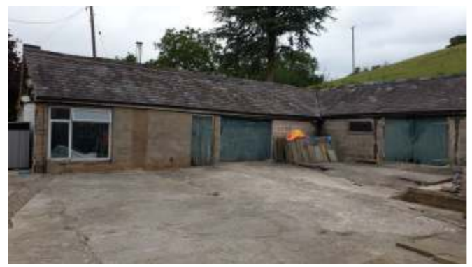
SOUTH AND PART WEST VIEW
