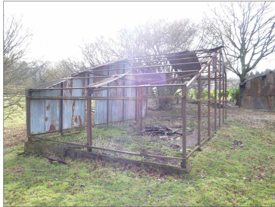
Photograph 2: Showing one of the former barns to be demolished.
