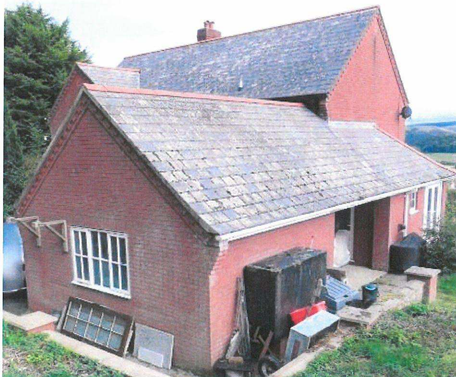
Photograph 4. Exterior. Left: parts of the Northwest elevation. Right: Southwest elevation.
