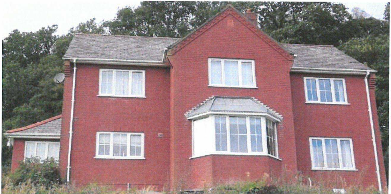
Photograph 2. Exterior. Southeast elevation.
