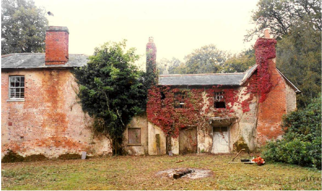
Photograph of the existing dwellinghouse (taken circa 1999)
