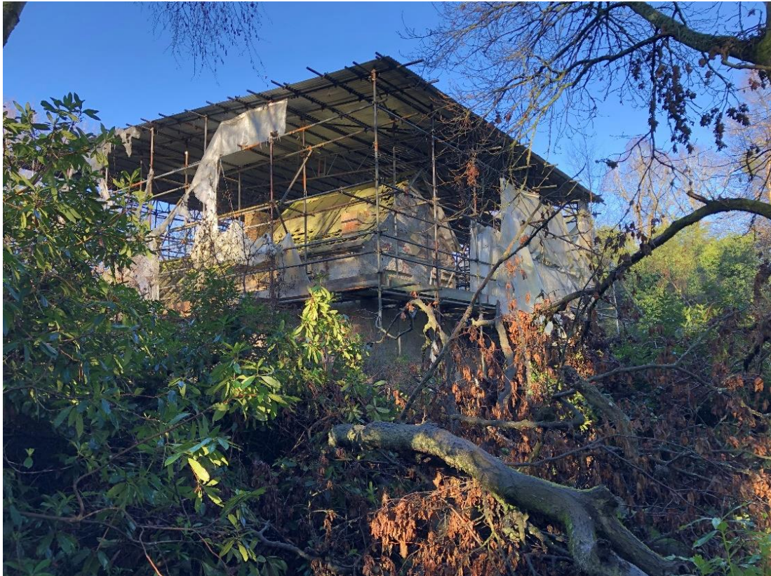
Photograph of the existing dwellinghouse (taken January 2022)
