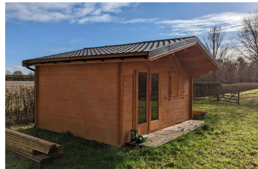
North West/South West Elevation - Photo - NTS (Unit 1)
