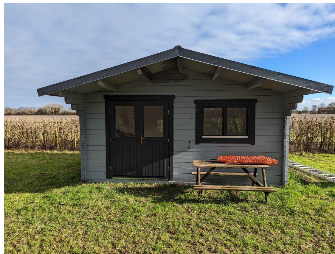
South West Elevation - Photo - NTS (Unit 2)
