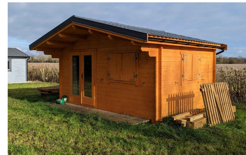
South West/South East Elevation - Photo - NTS (Unit 1)
