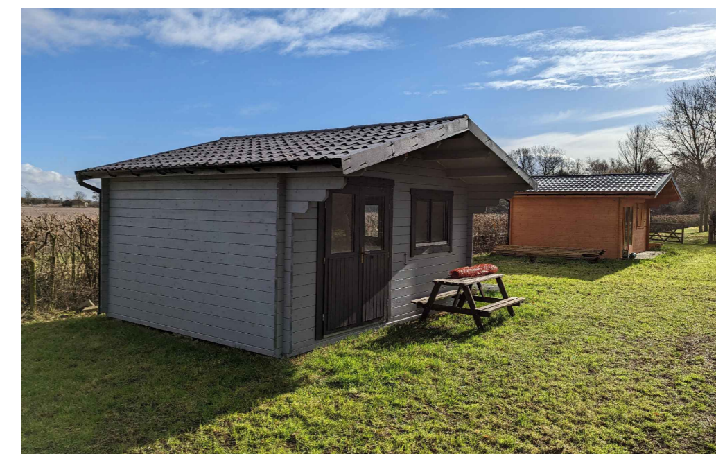
North West/South West Elevation - Photo - NTS (Unit 2/1)
