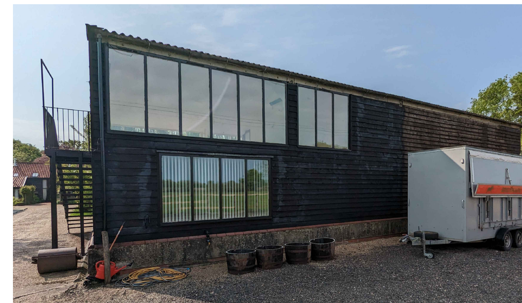
Existing North West Elevation Photo (NTS)
