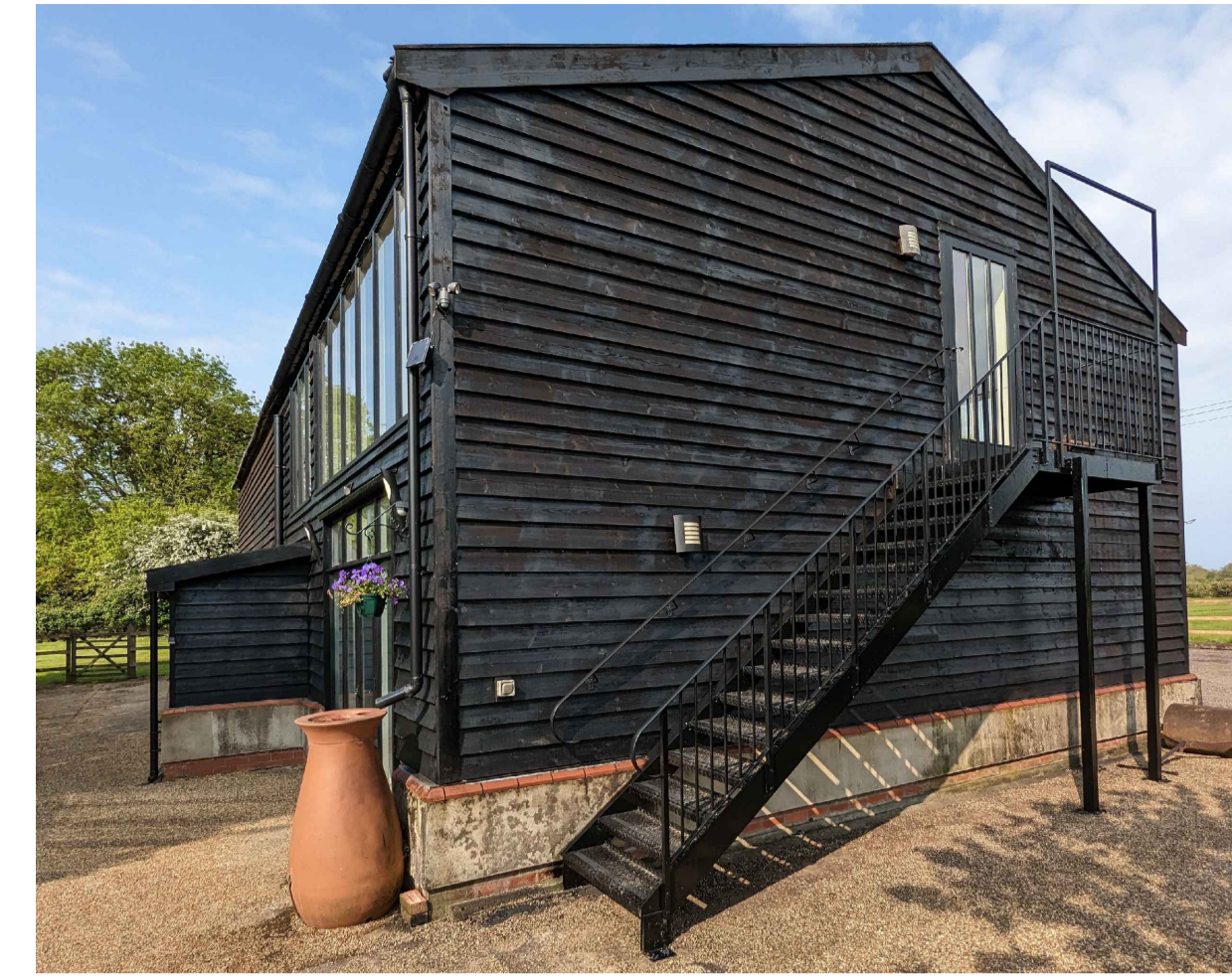
Existing NE Elevation Photo (NTS)
