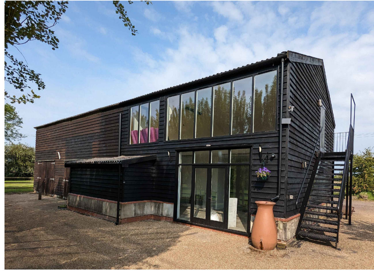
Existing SE/NE Elevation Photo (NTS)
