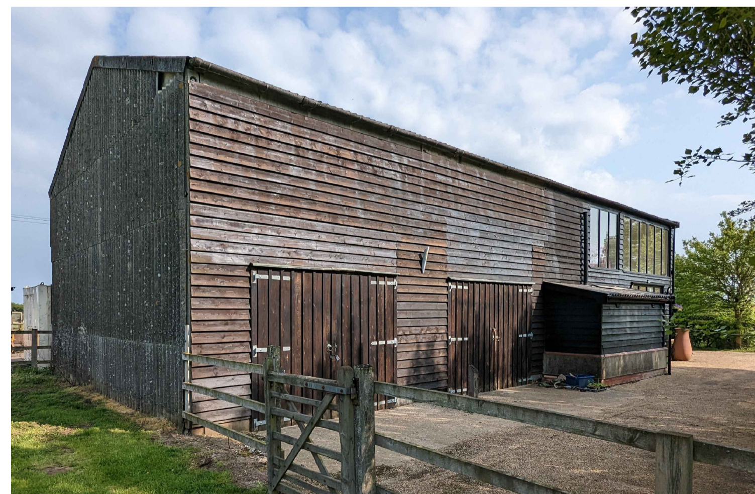
Existing SE/SW Elevation Photo (NTS)
