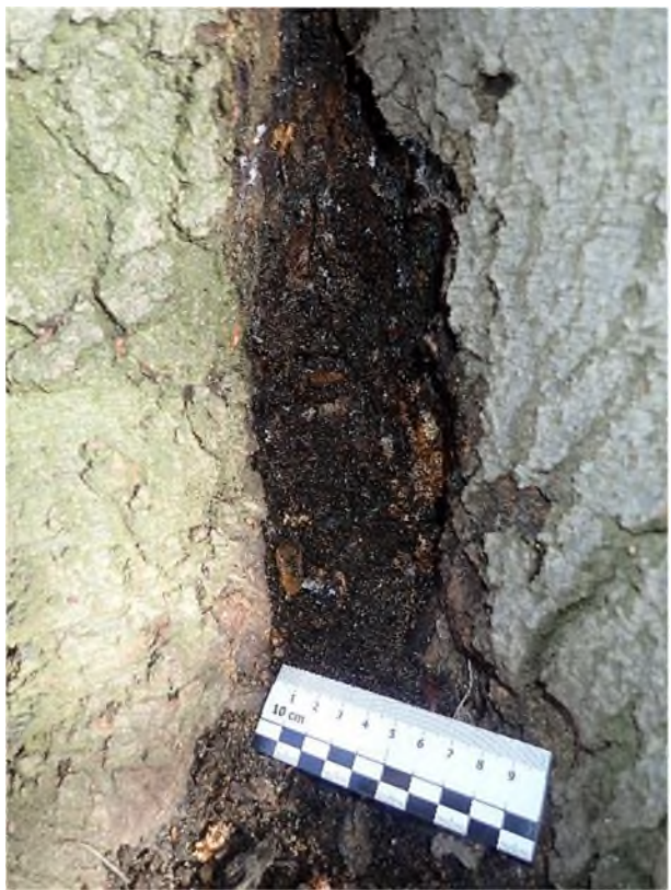
Detail of Honey Fungus decay
