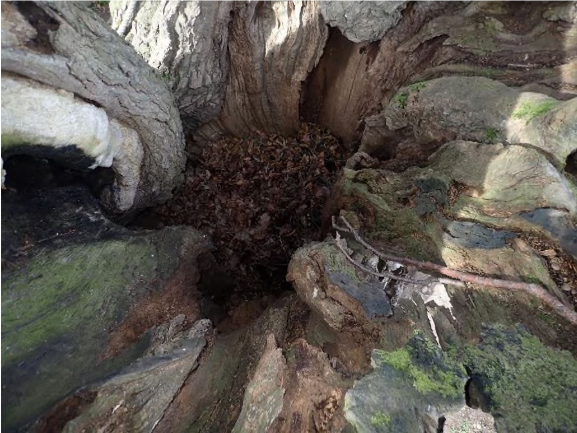
Looking down into the hollow upper stem
