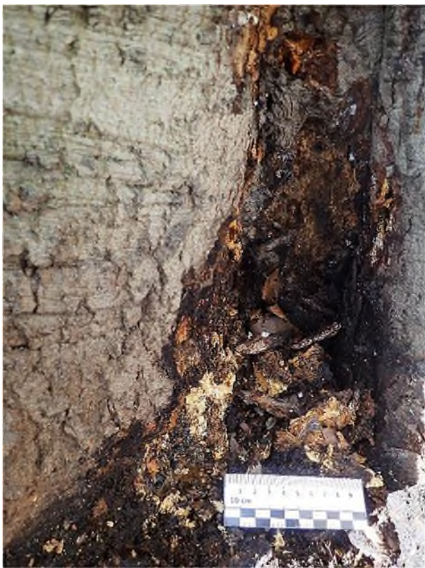
Detail of Honey Fungus decay
