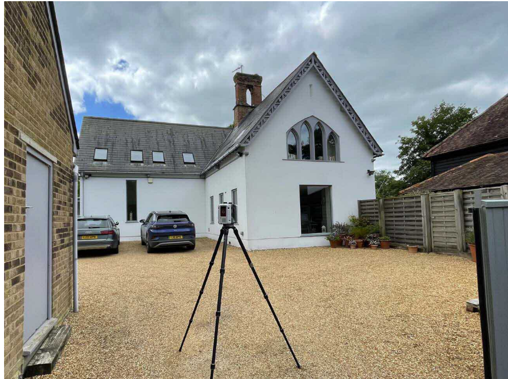
Figure Desc. View of the principal elevation
