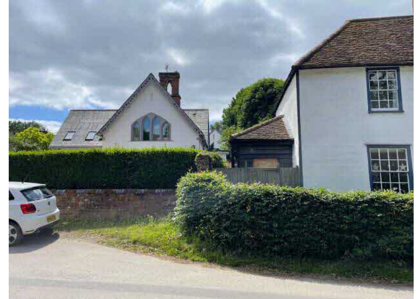
Fig Desc. Neighbouring property to the Old School
