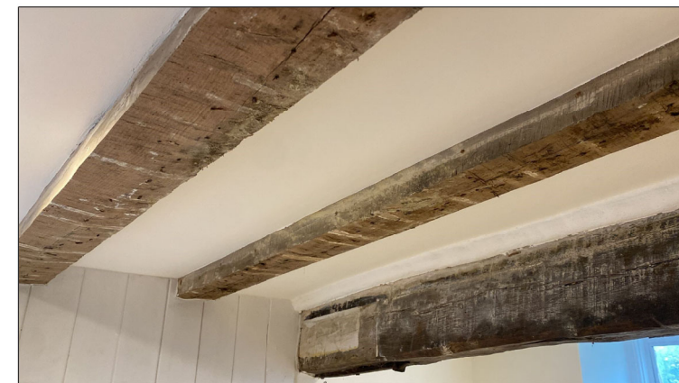
Photo of exposed beams
