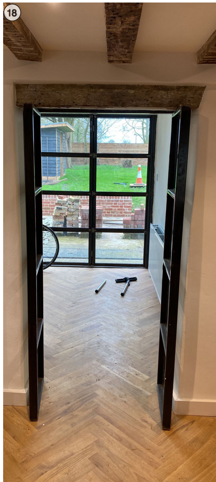
Photo of Current condition
