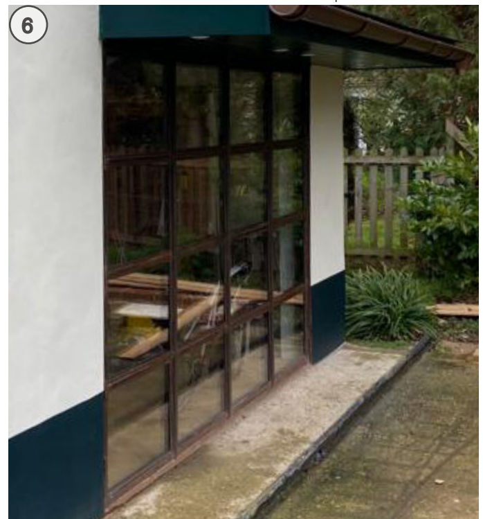
Photo of current condition around C20 SE Sloped extension
