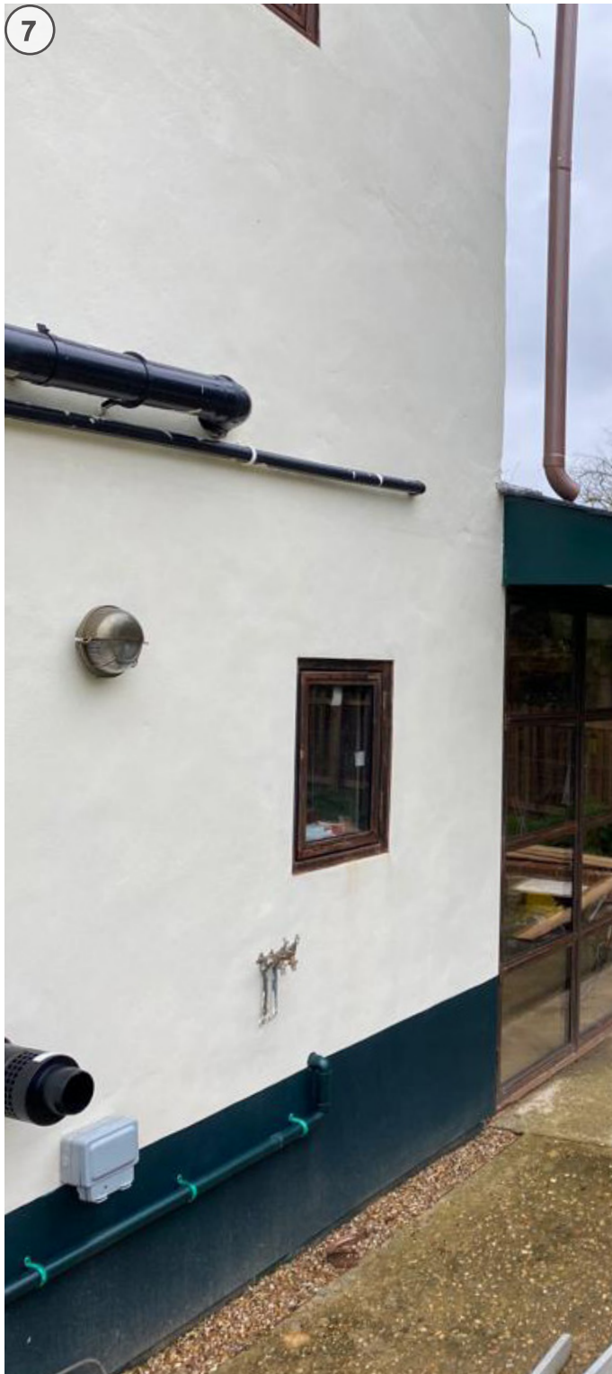
Photo of current condition
