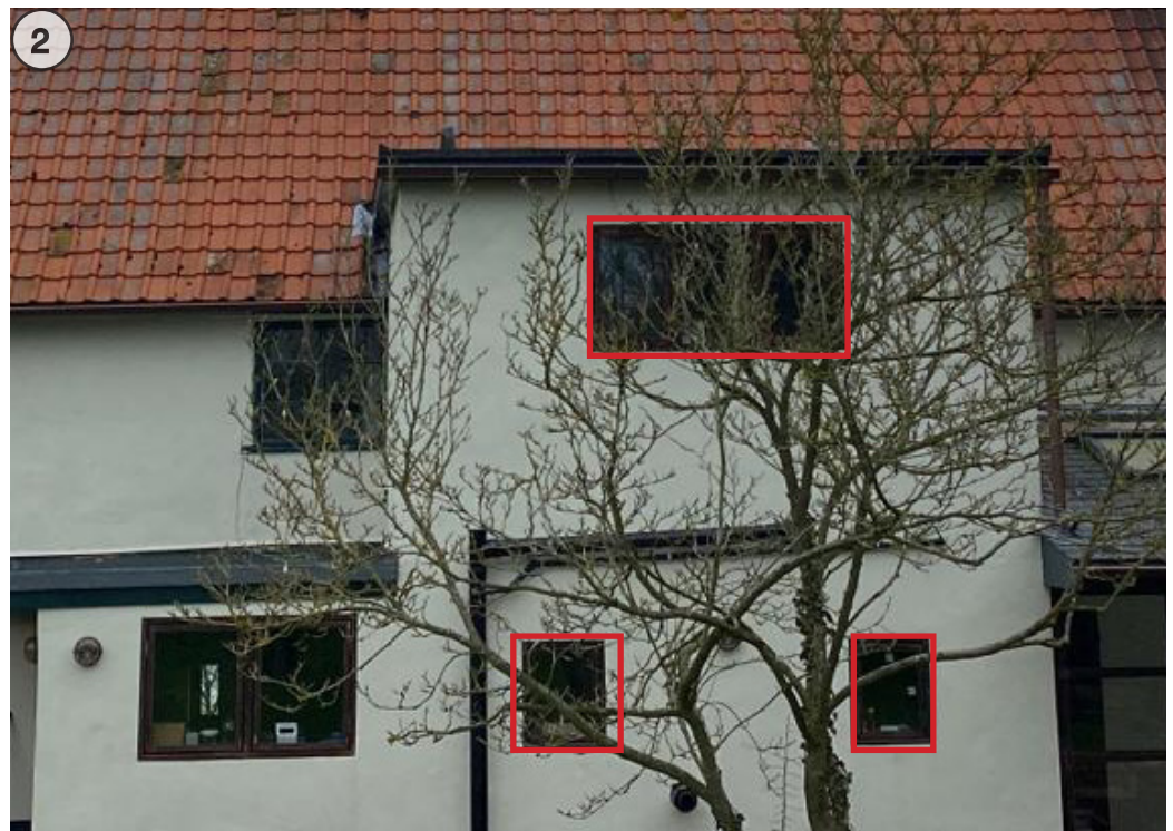
Photo of current condition
