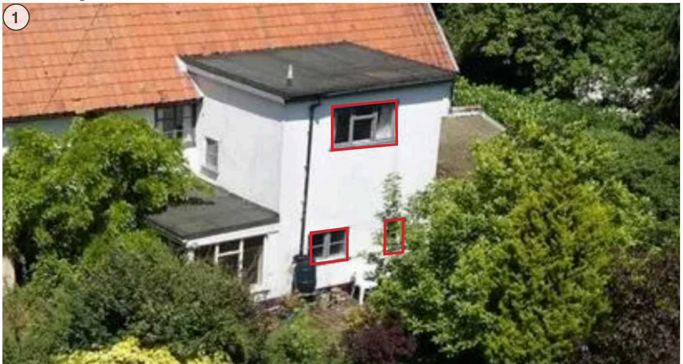
Photo of current condition
