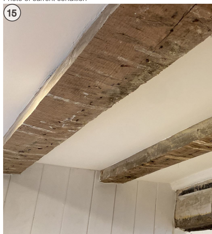
Photo of current condition
