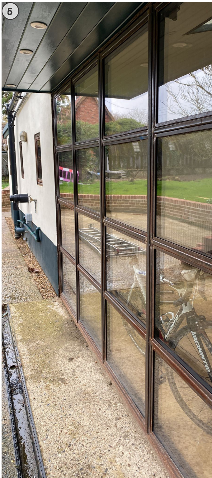
Photo of current condition
