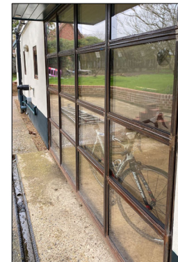
Steel Frame and surround crittall style windows with double glazing inserts
