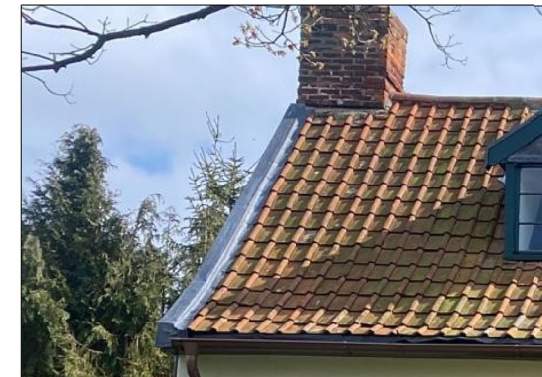
Replacement lead flashing - like for like to existing
