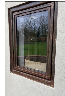
Steel Frame and surround crittall style windows with double glazing inserts
