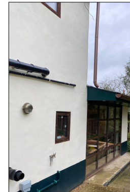
Lime mortar 5-1-1 mix used to re-render the modern extension to the south of the property
