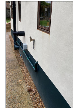
Lime mortar 5-1-1 mix used to re-render the modern extension to the south of the property
