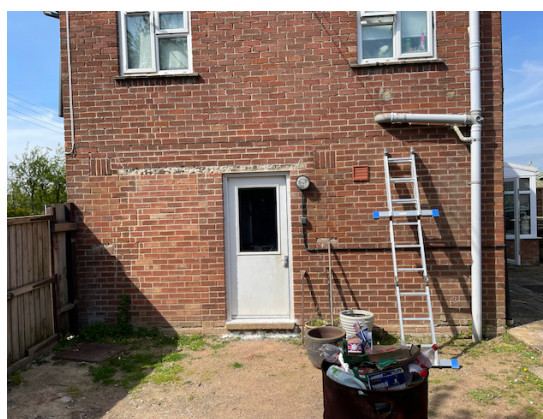
South elevation where the extension is to be built
