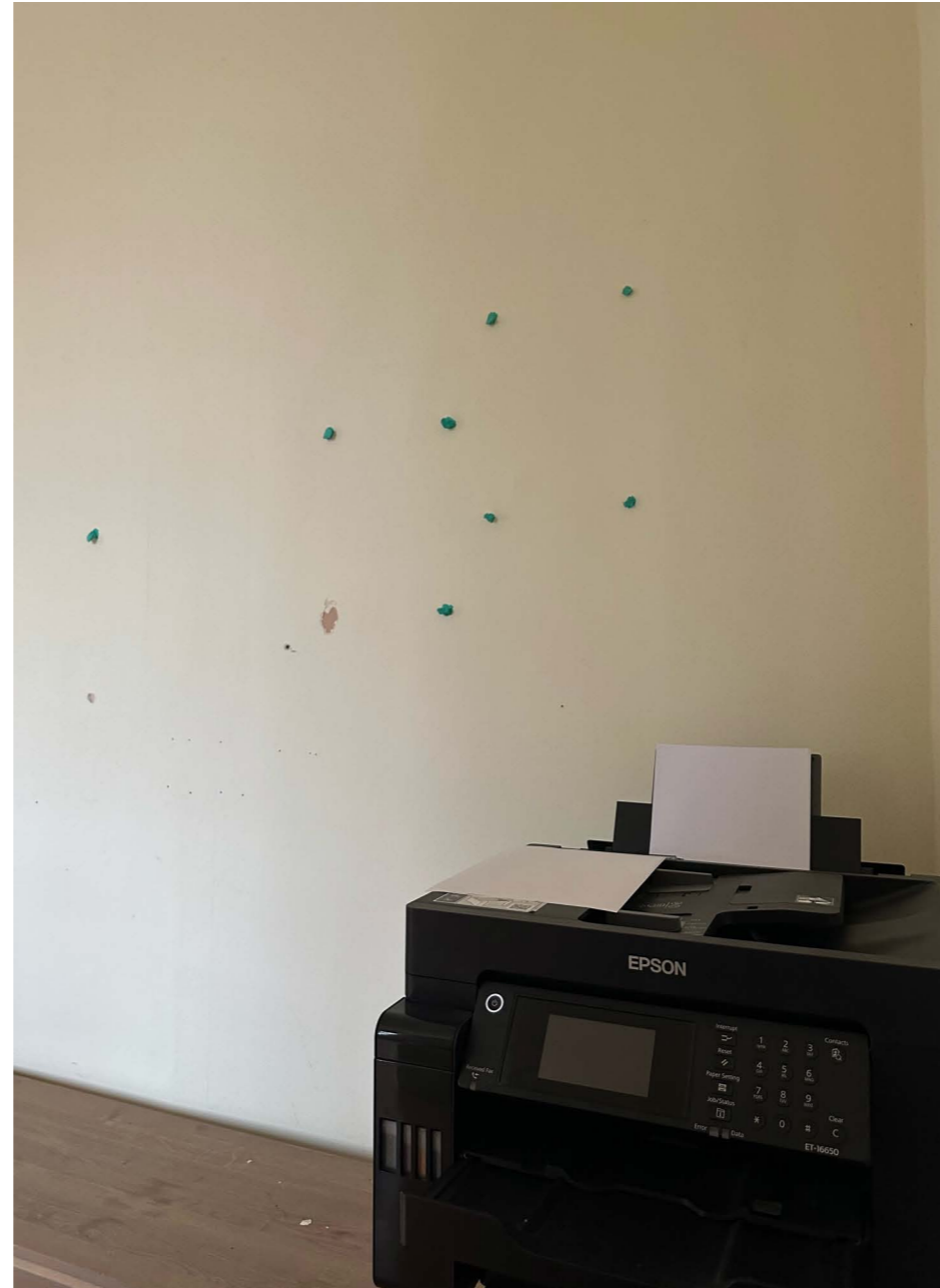
View of existing living space showing wall to be removed. No original architectural detailing visible.
