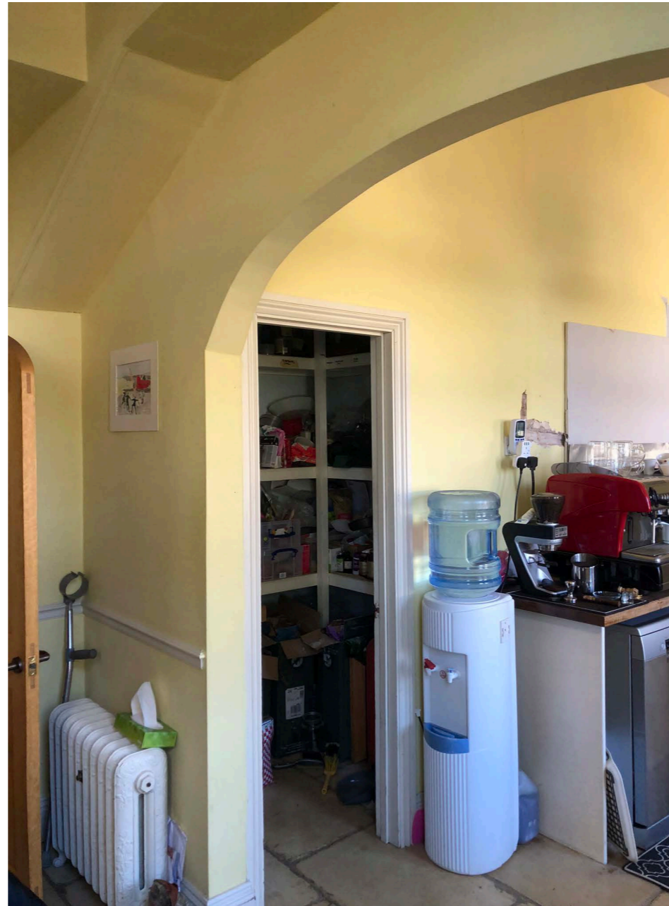
View of existing kitchen showing wall to be removed.
