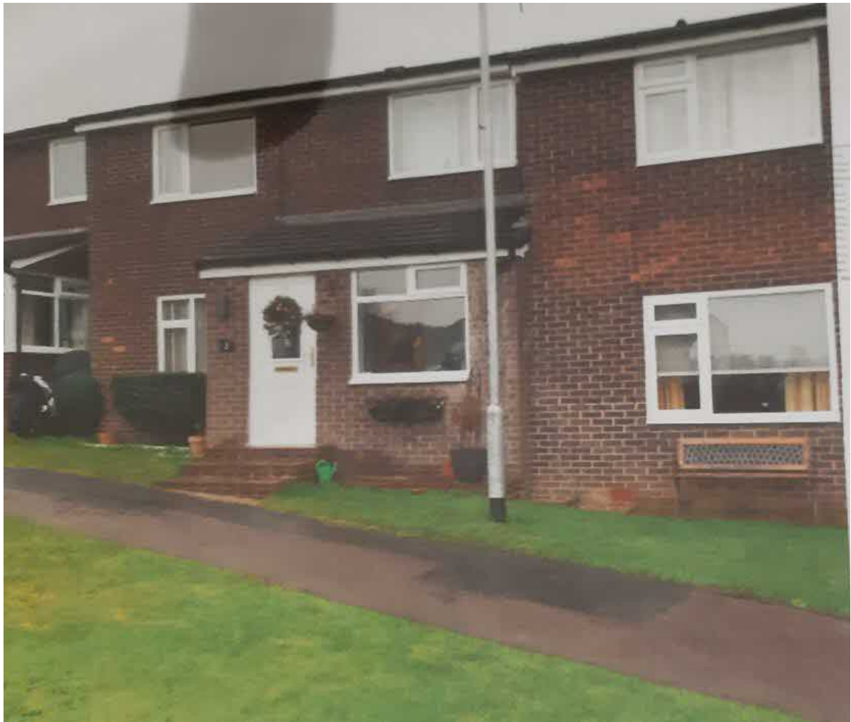
Figure 2 – Neighbours Property No:3 Addycombe Crescent
