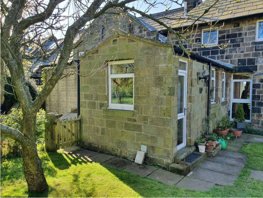
Image 2 – Existing original extension (rear)
