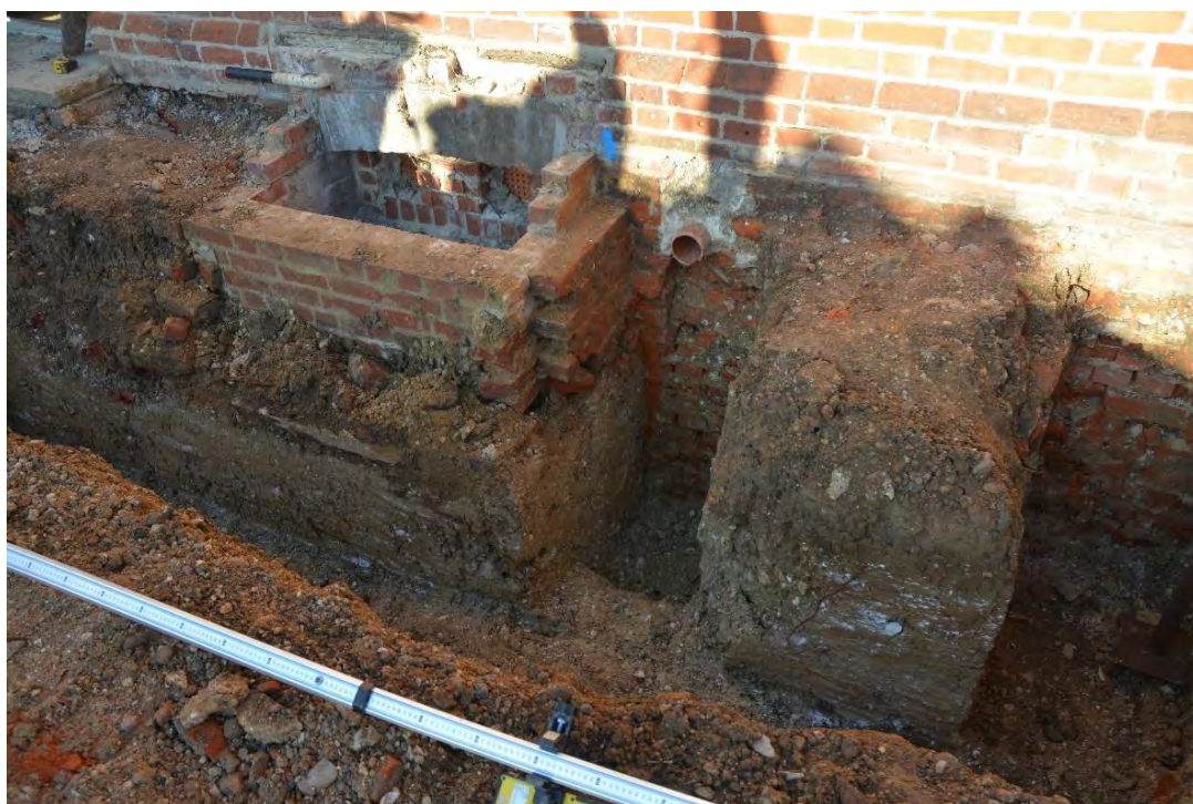
Plate 16: Eastern foundation trenches, including view of possible coal chute. View west.
