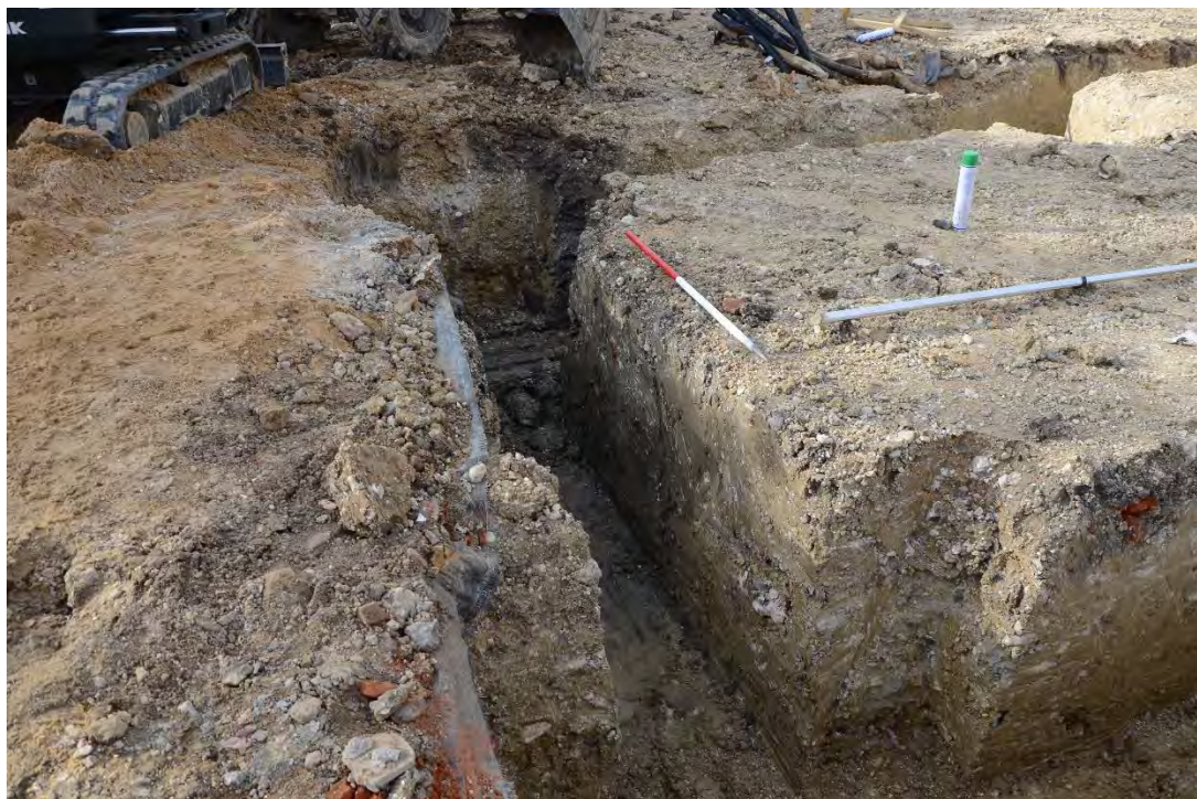
Plate 13: Oblique view of possible moat [4] being excavated. View north-west.
