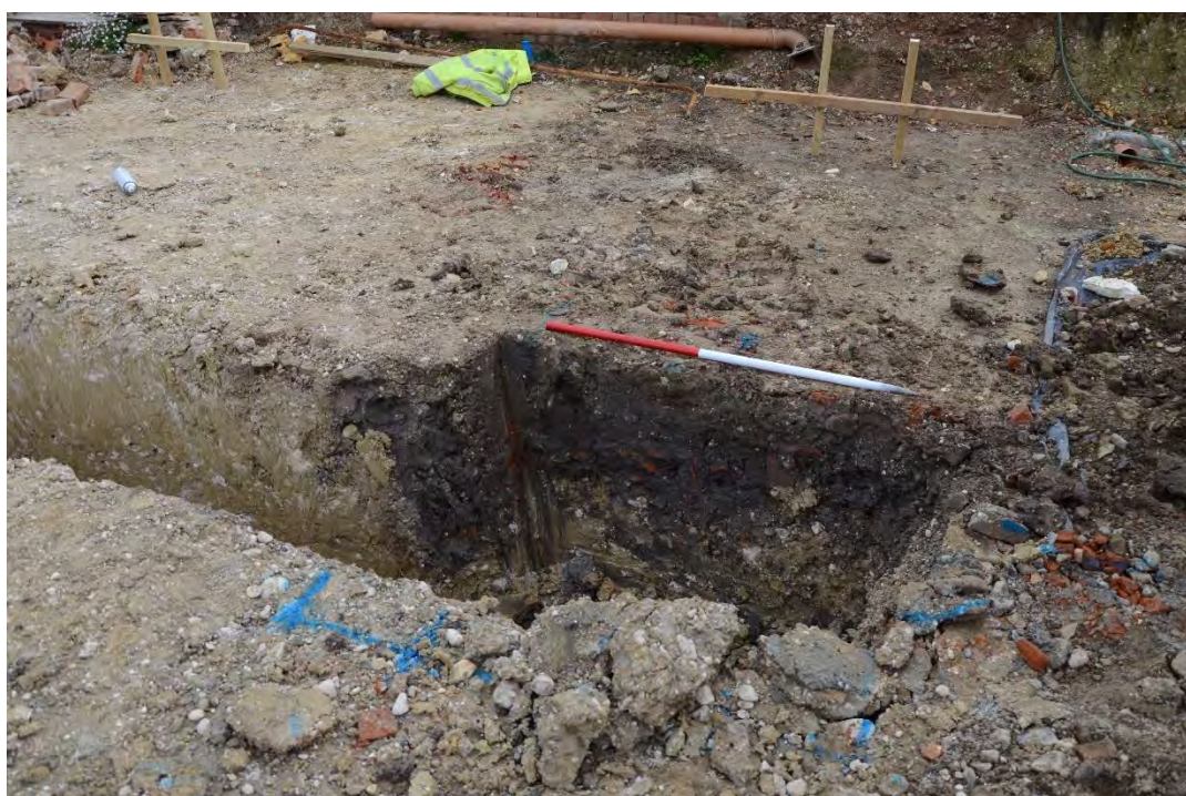
Plate 14: Structure (6) and feature [15]. View east.
