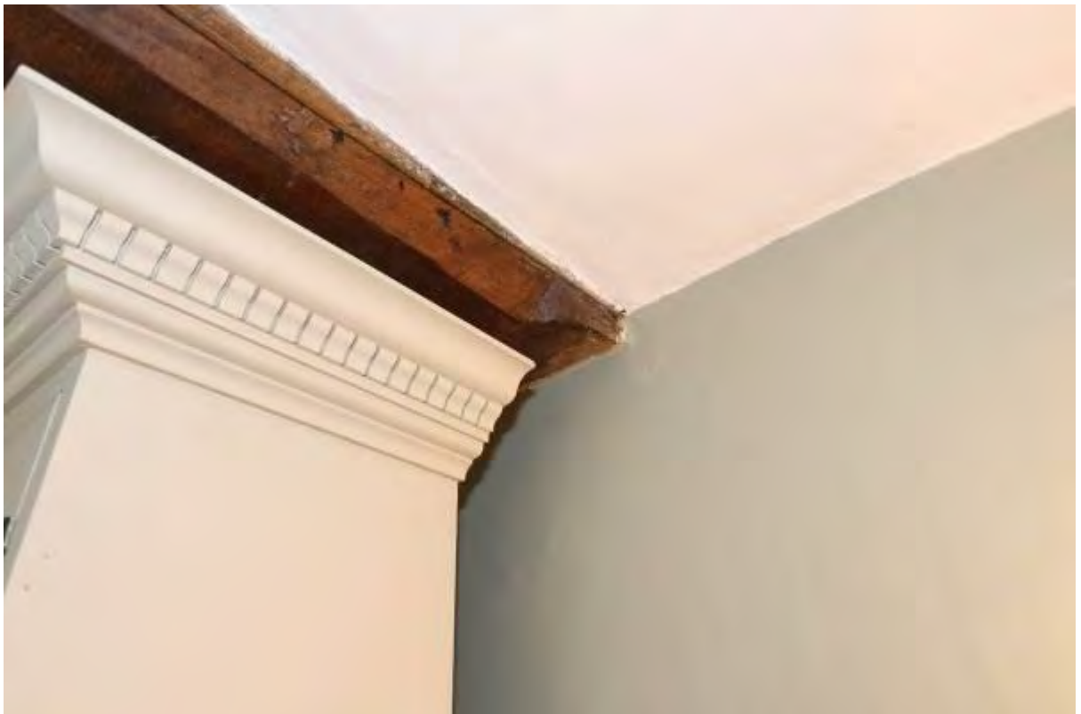
Plate 12 Axial beam with stopped chamfer (G1)
