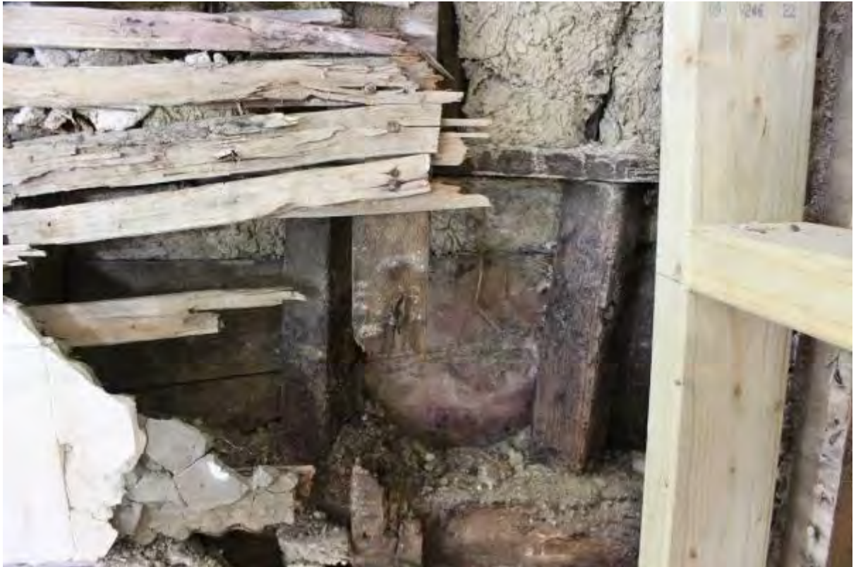
Plate 65 Detail of in-situ diamond-set mullions of mullioned window and later blocking
