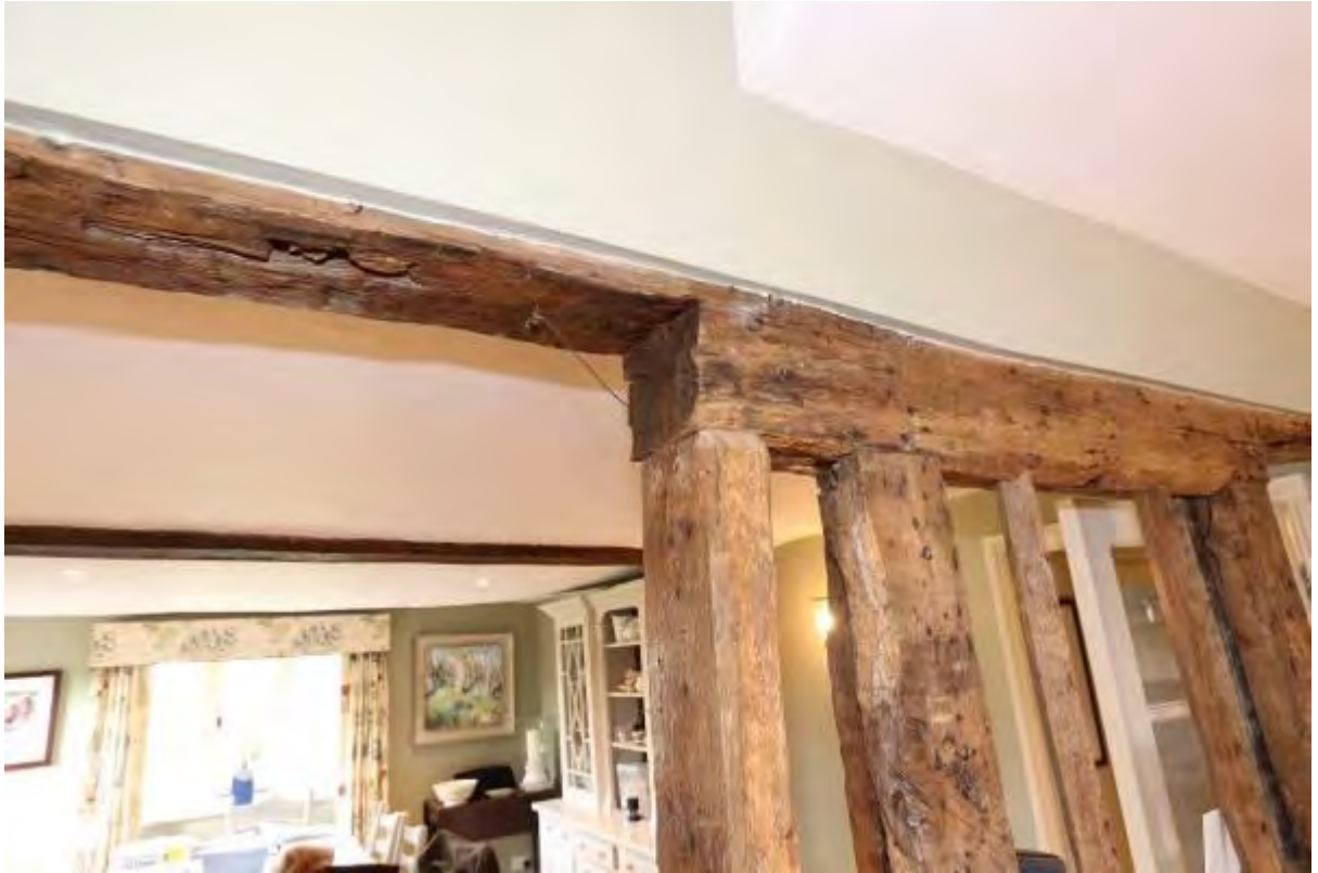
Plate 15 Cut away of former doorway (south), looking west
