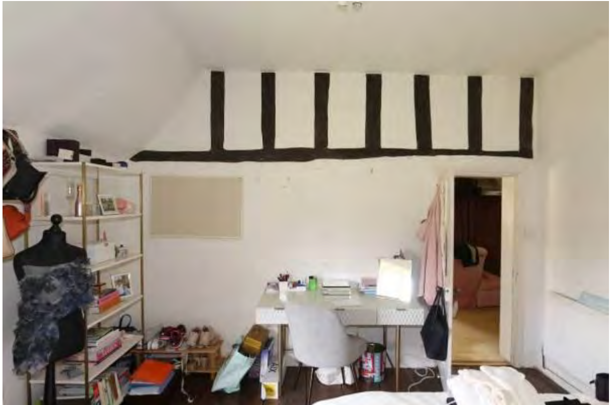
Plate 34 Bedroom (F2), showing studwork of end wall
