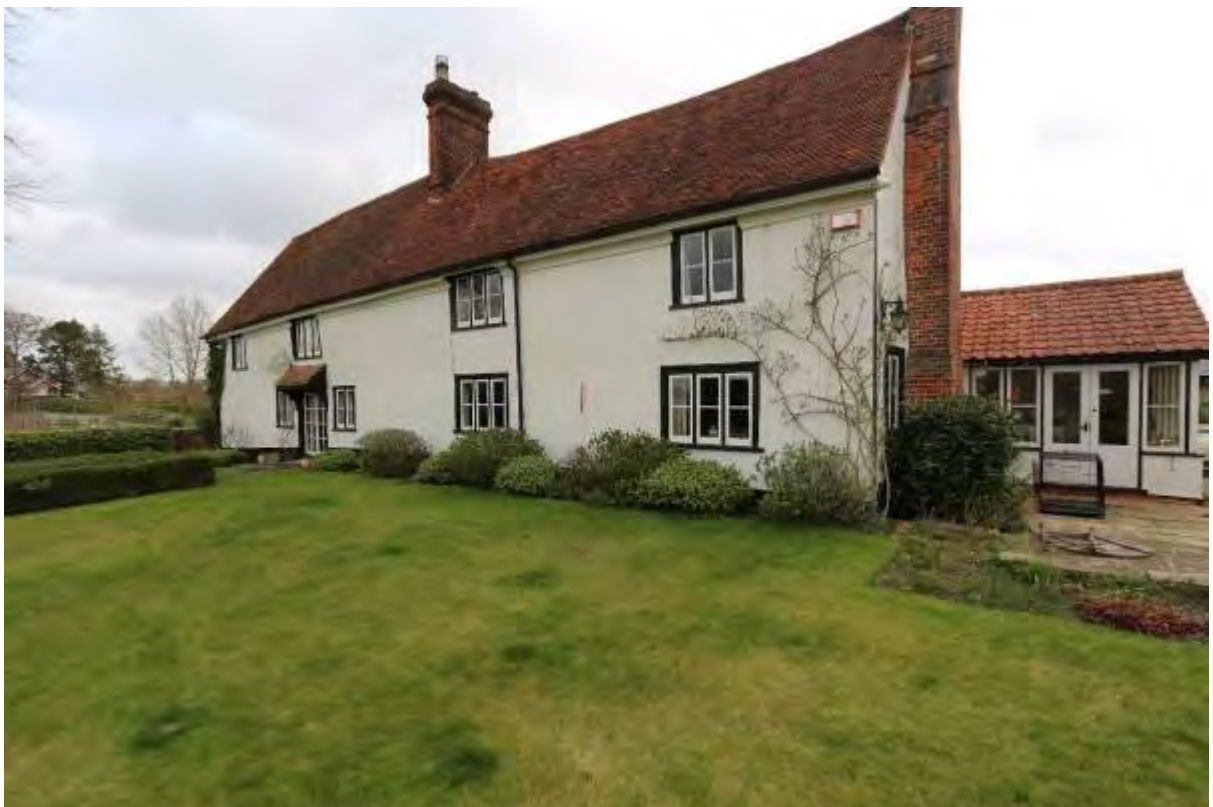
Plate 2 Western Elevation looking north-east
