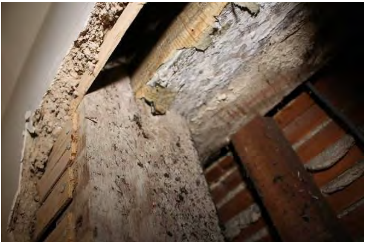
Plate 54 Wallpapered-over wall plate and softwood stud, looking east from (F5)
