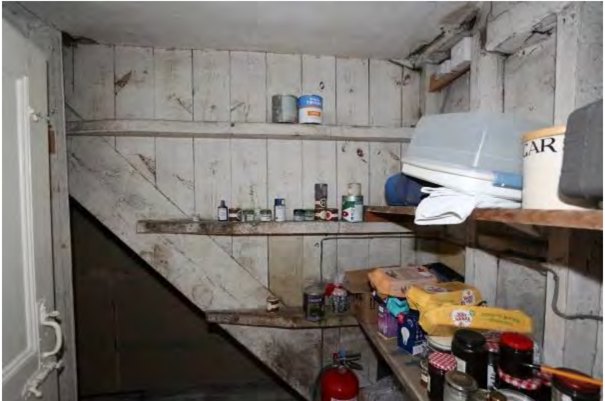
Plate 23 Stair (G12) from basement, showing timber stud wall (right)
