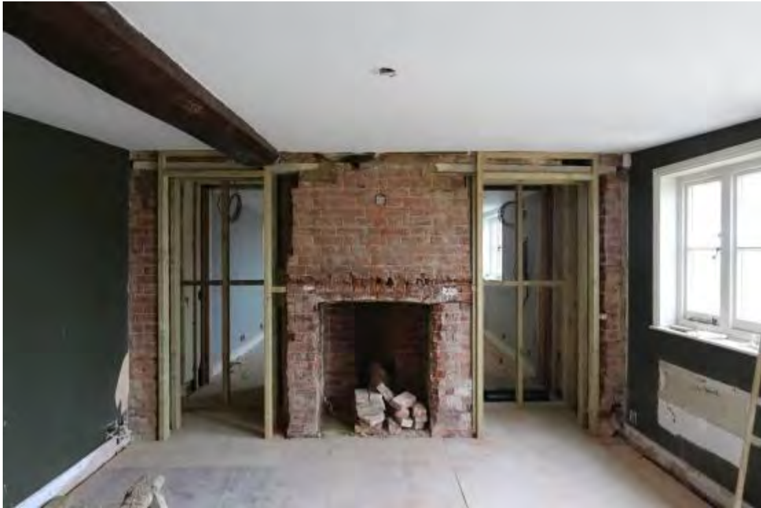
Plate 71 Rebuilt fireplace/stack in (G8)
