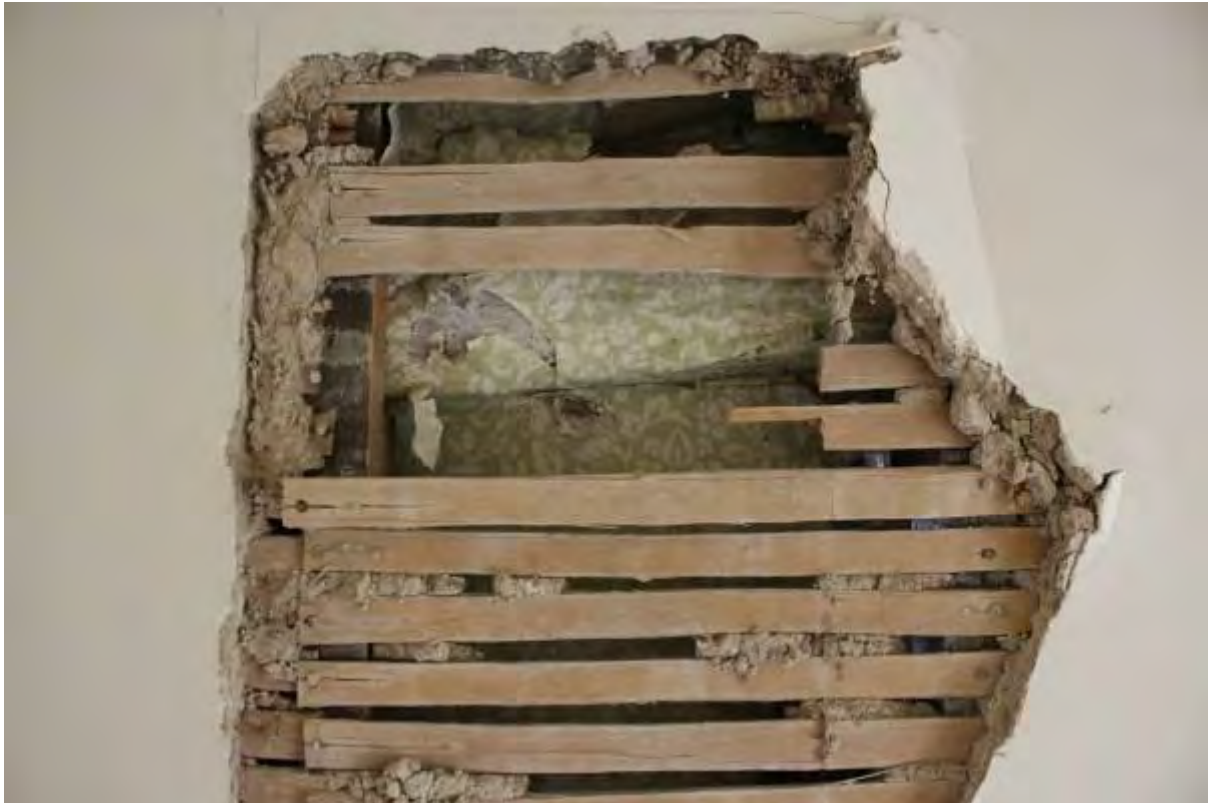
Plate 55 Wallpapered-over wall plate seen in in opening (C)
