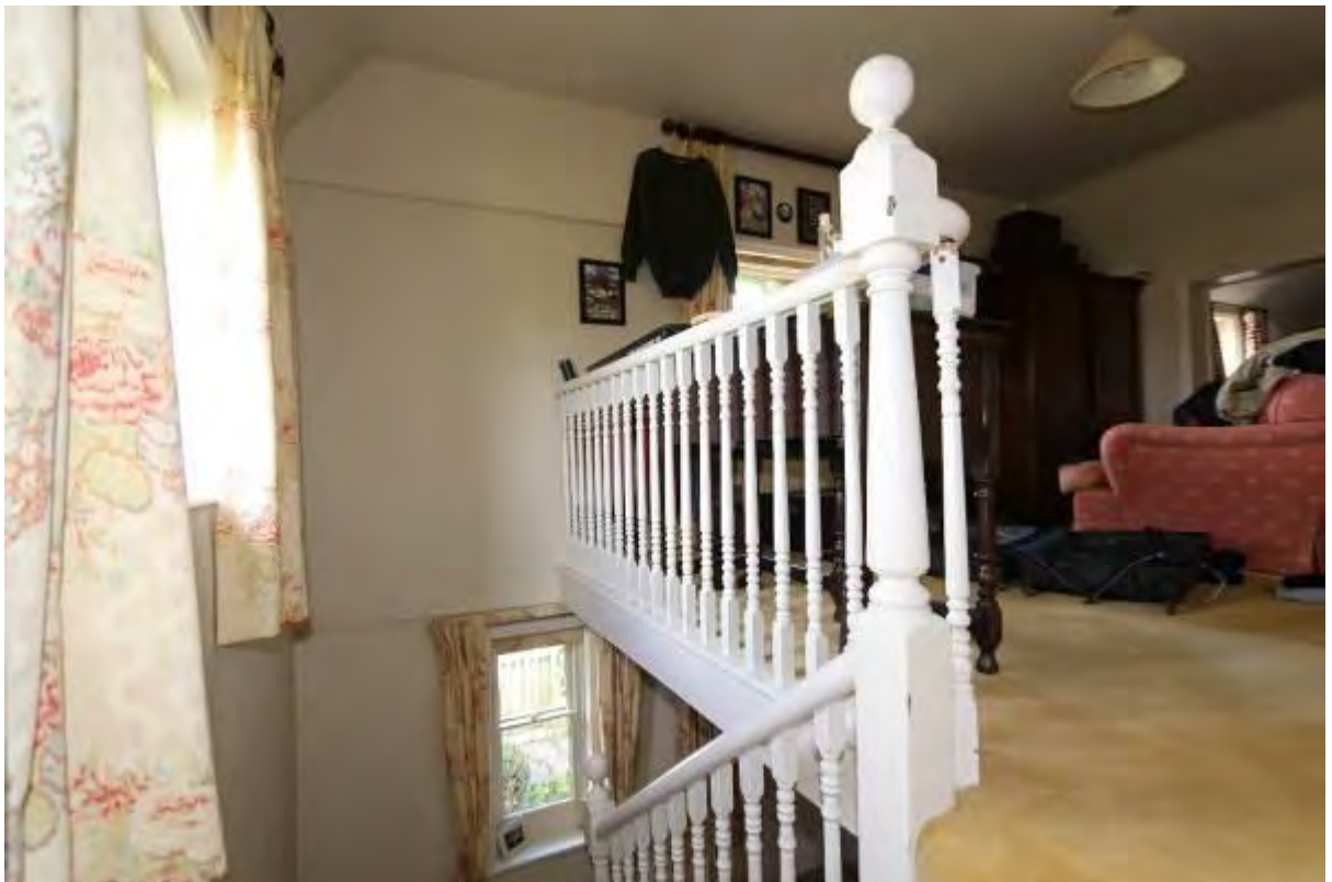
Plate 31 Stair banister to first floor landing (F1)
