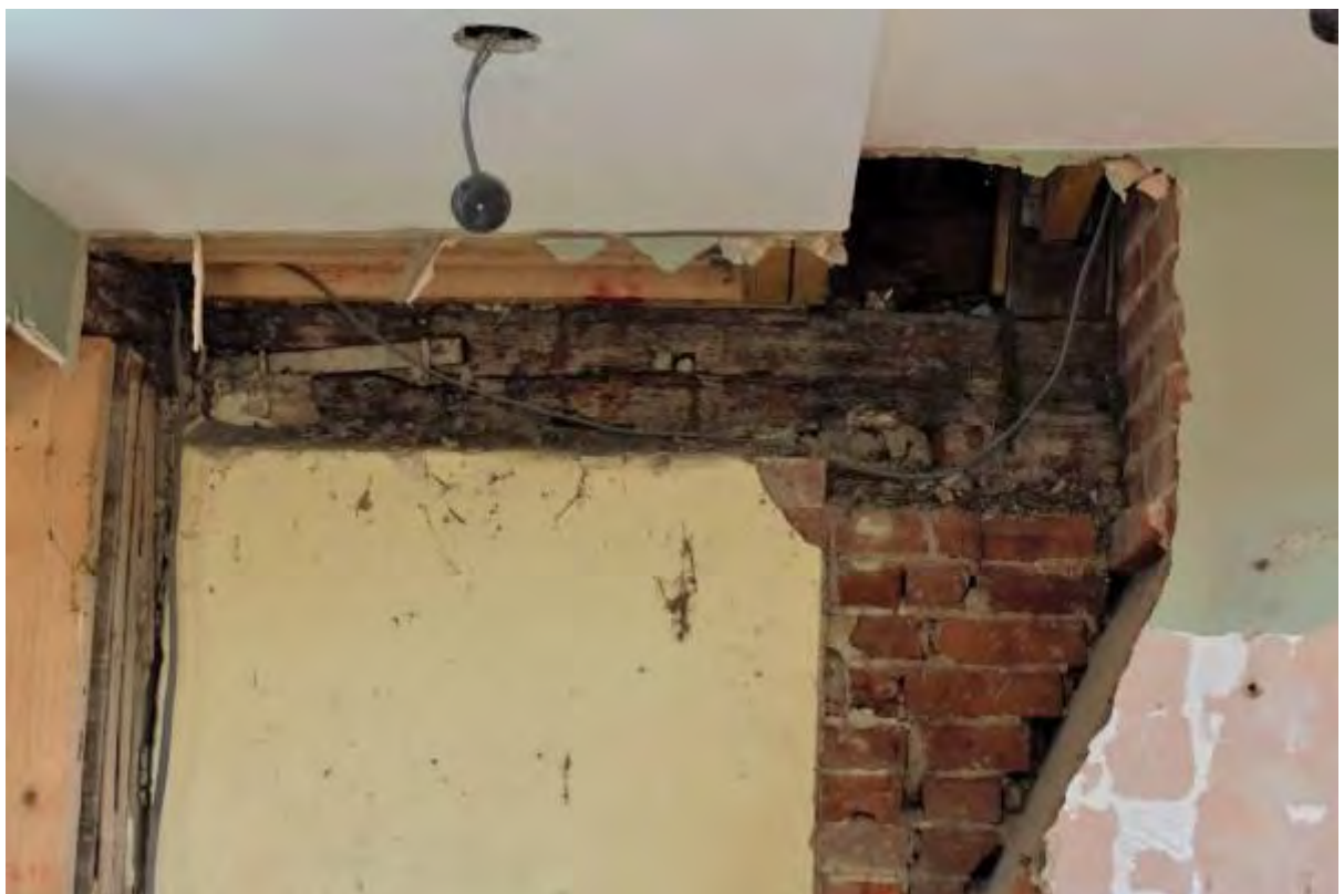
Plate 52 Southern mid rail to stair turret, looking north
