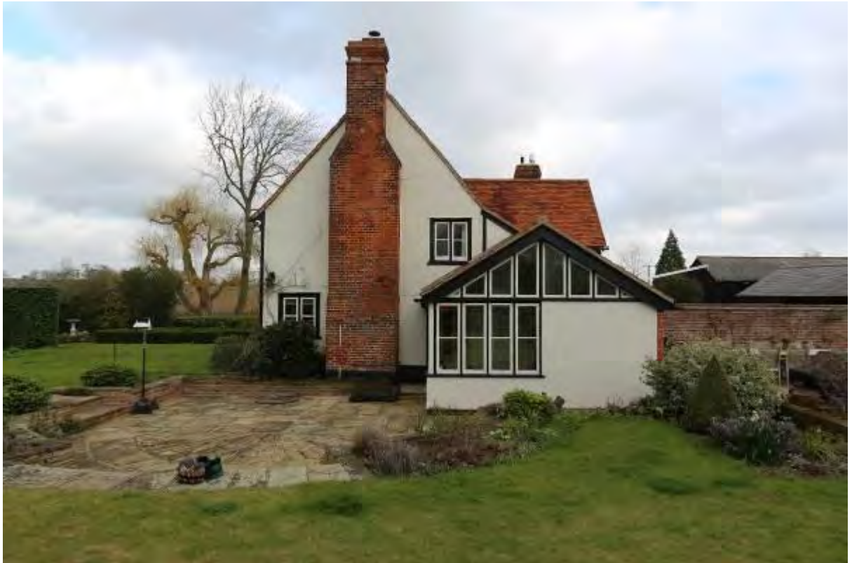
Plate 9 Southern Elevation looking north
