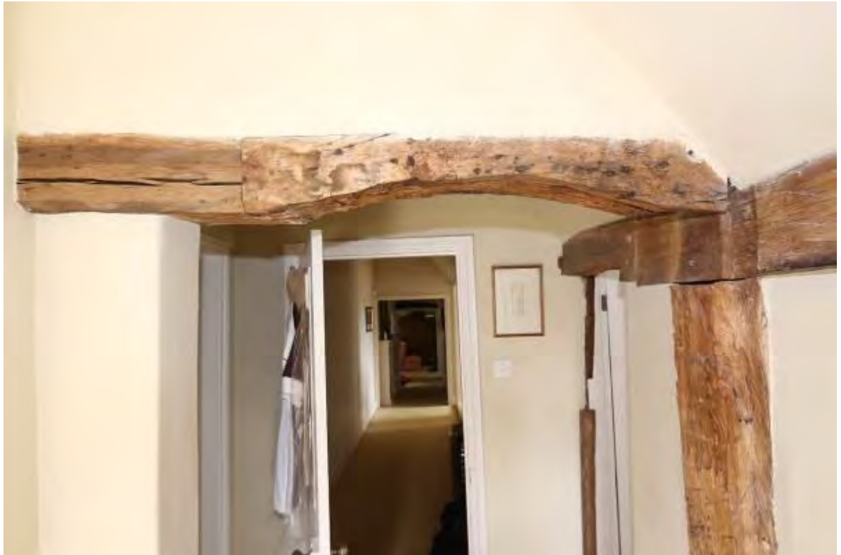
Plate 38 Doorway cut into soffit of tie beam (F4) looking north
