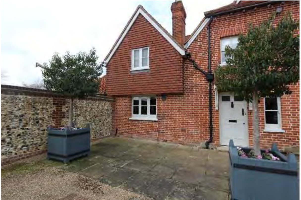
Plate 5 Eastern Elevation, southern bays, looking south-west
