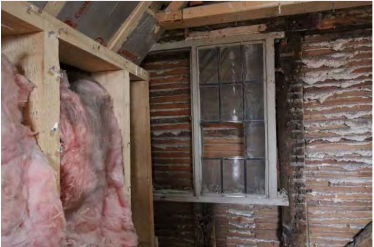
Plate 69 Detail of former casement window to bedroom (F4)
