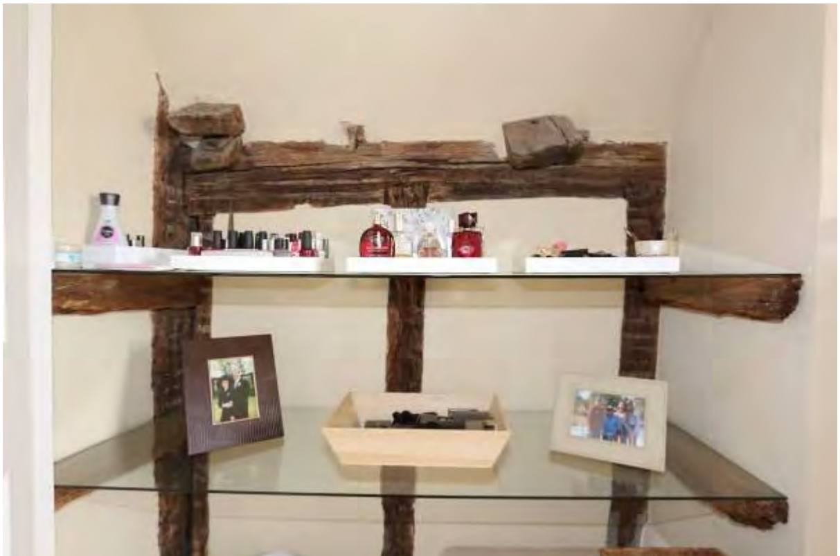
Plate 41 Extant timber studwork and rafter feet in (F10), looking north
