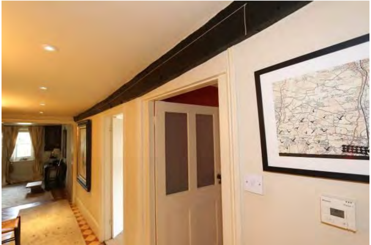
Plate 24A Extant mid-rail in passage (G4) and part glazed door into (G6)
