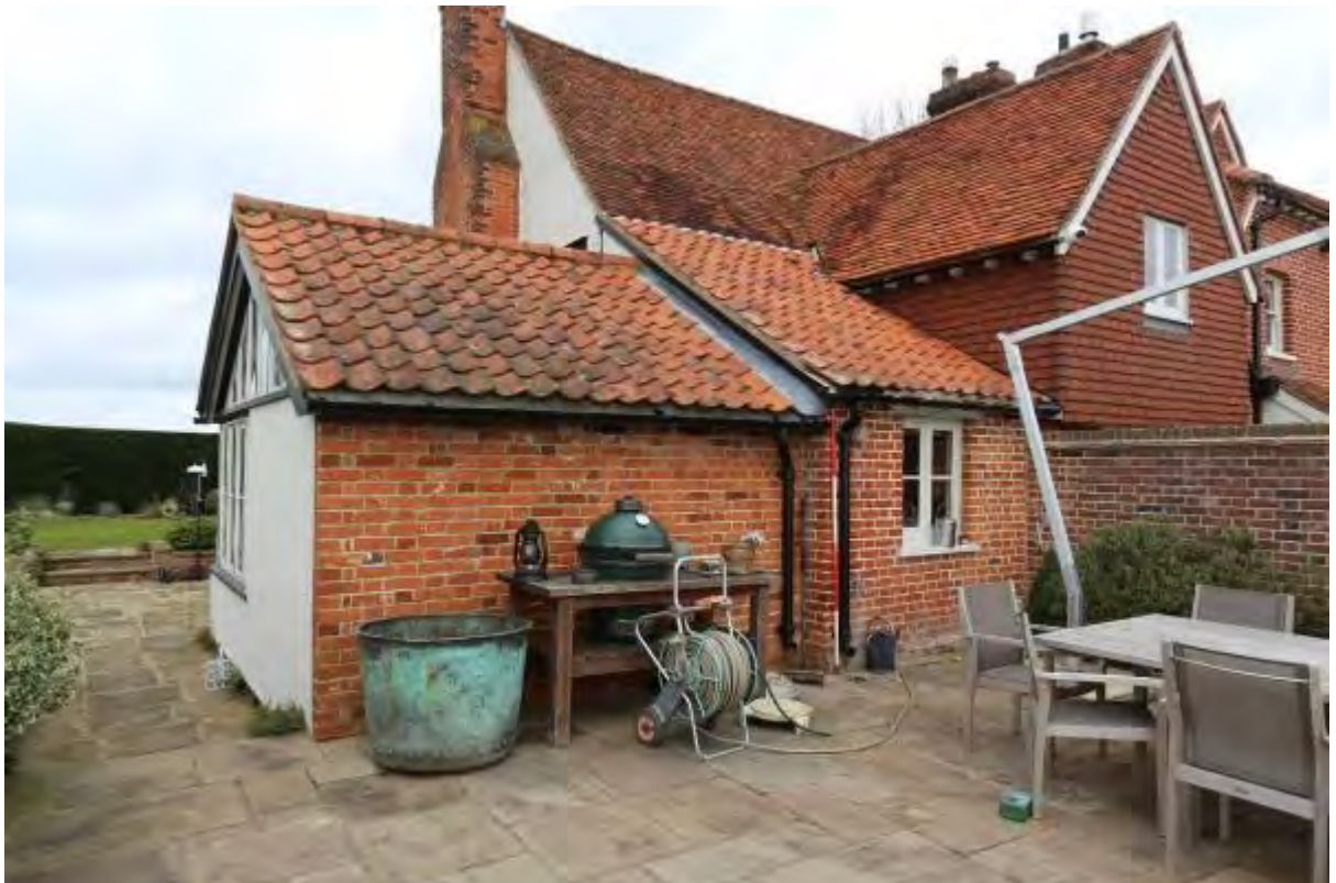
Plate 6 Eastern Elevation, southern bays and extension, looking north-west
