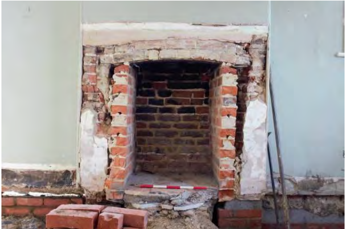
Plate 51 Rebuilt fireplace in (G1), looking north
