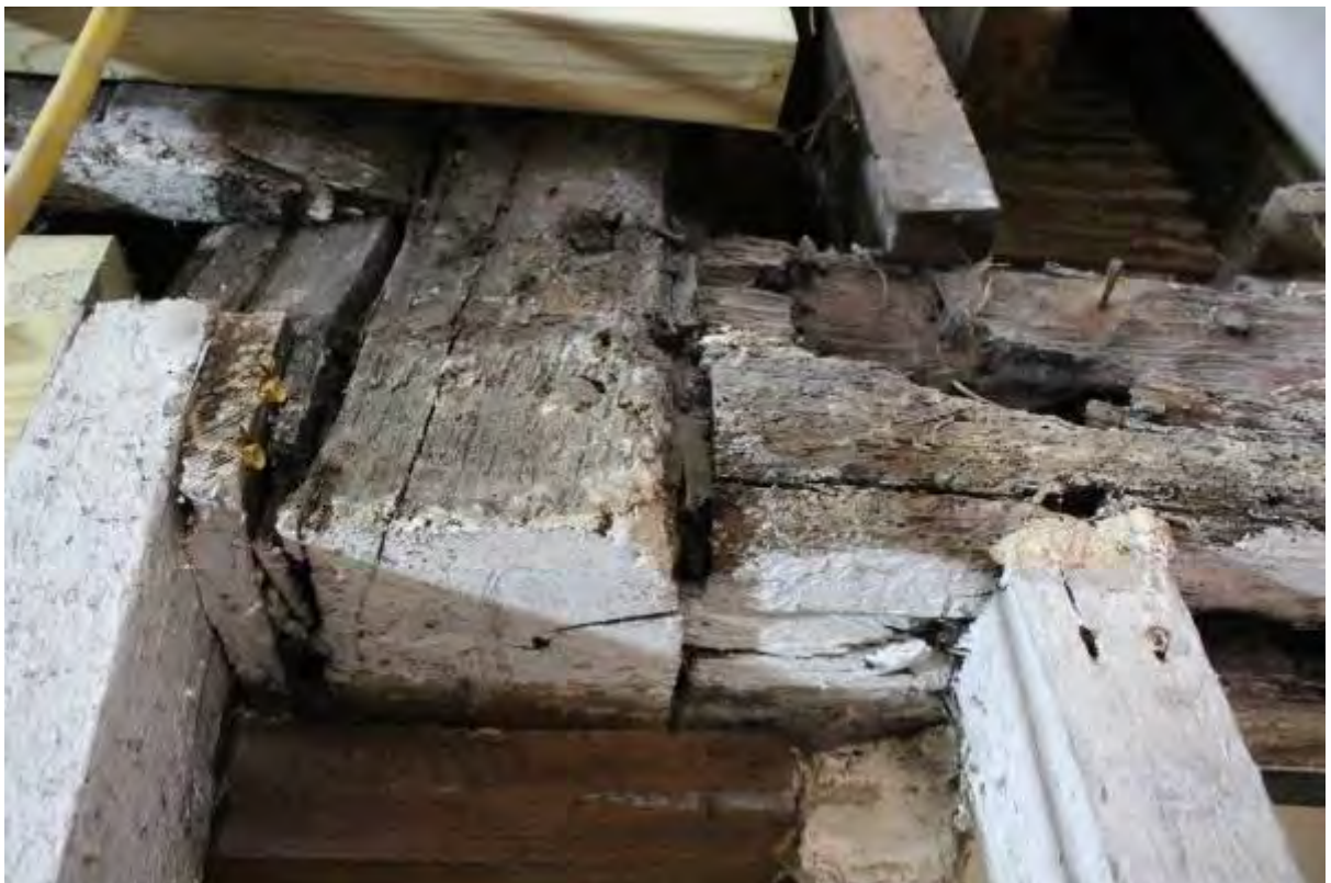
Plate 62 Cut off storey post
