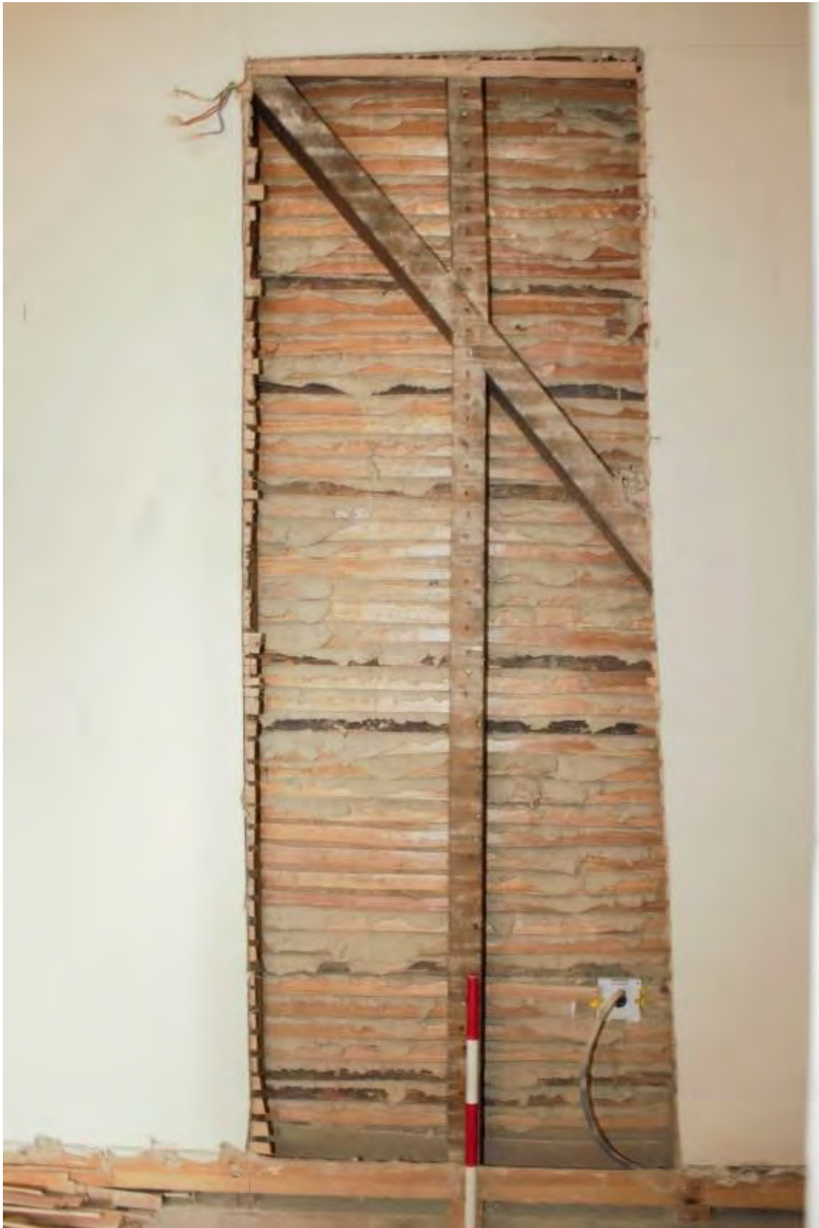
Plate 50 Opening A between dining room (G8) and passage (G4)
