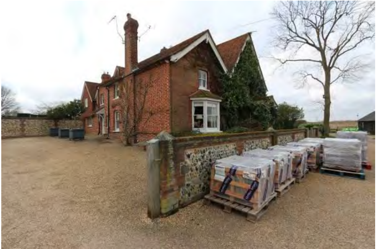
Plate 7 Northern and Eastern Elevations looking south-west
