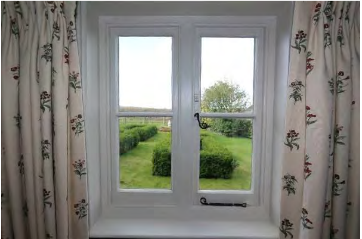
Plate 28 Detail of inserted casement window (G8)
