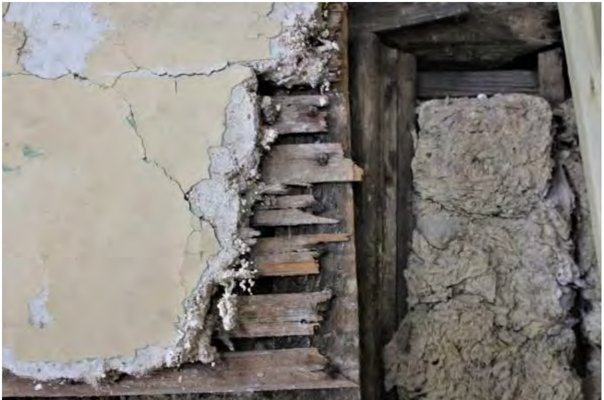
Plate 66 Inserted moulded mullion of smaller window and later blocking-in
