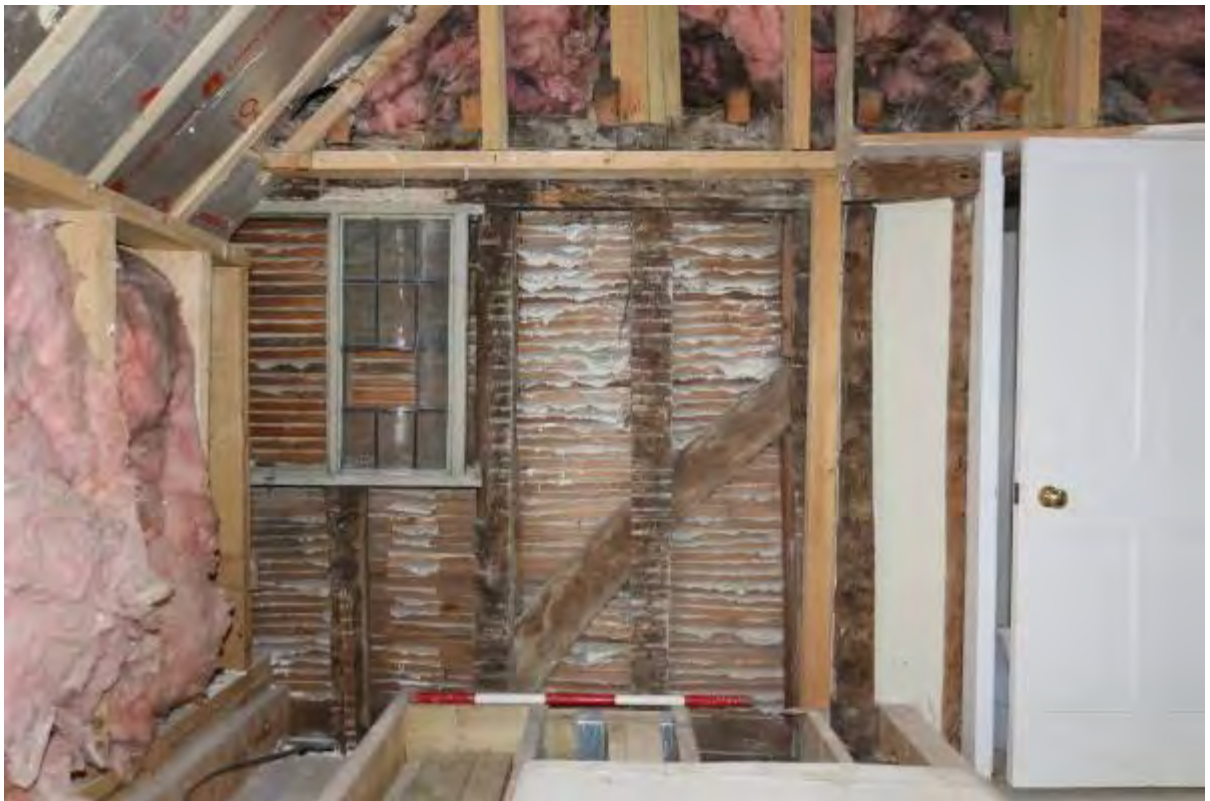
Plate 68 Historic wall between Bedroom (F4) and ensuite (F10)
