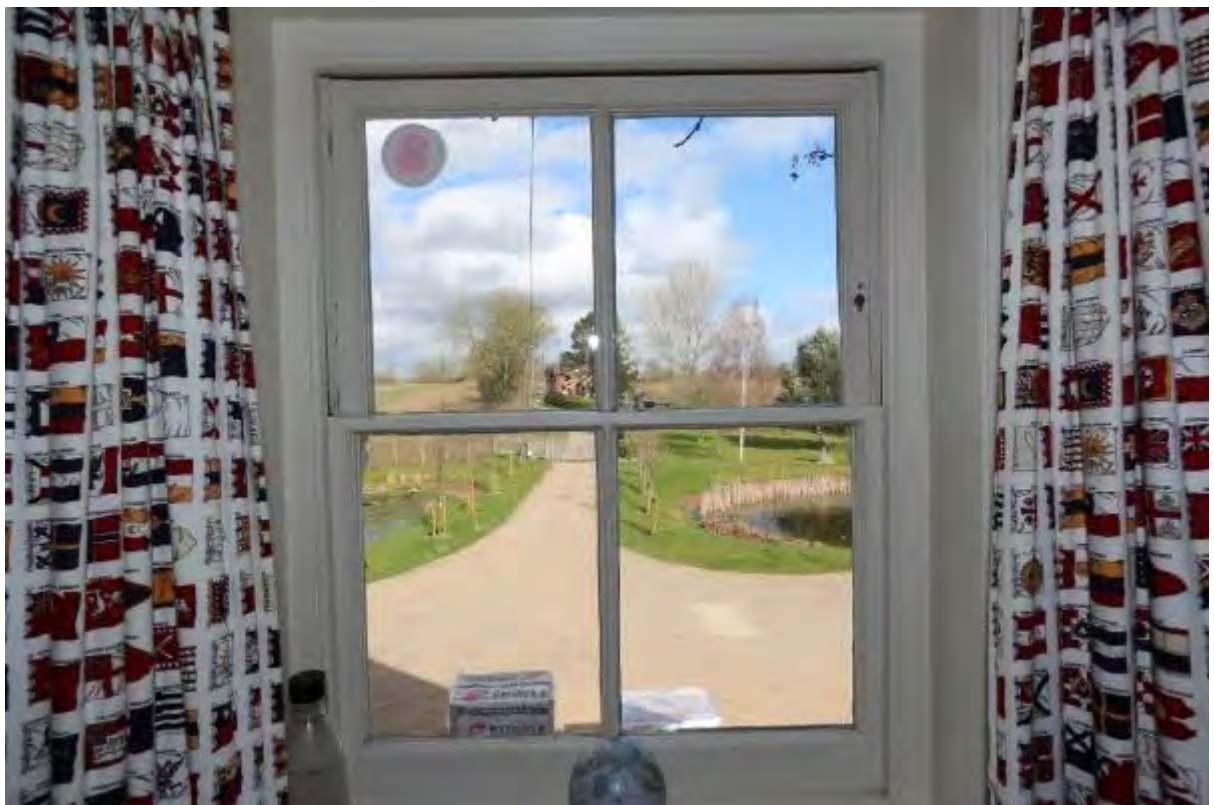
Plate 49 Sash window in (F6) looking north
