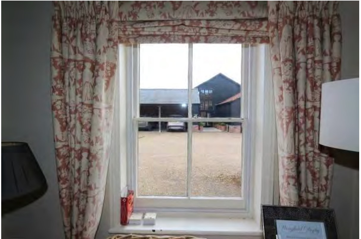
Plate 26 Detail of sash window (G7)
