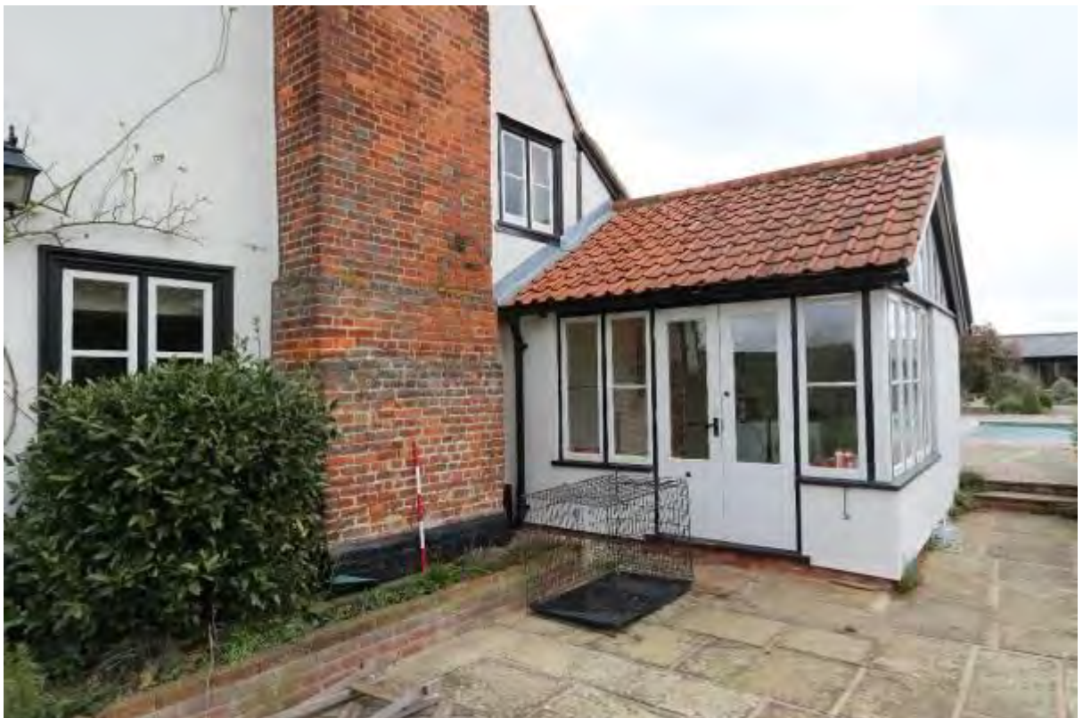
Plate 10 Garden Room looking east
