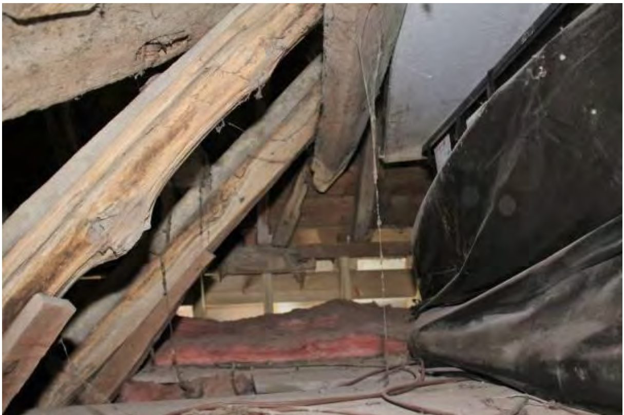
Plate 70 Historic side purlin roof surviving over former stair turret
