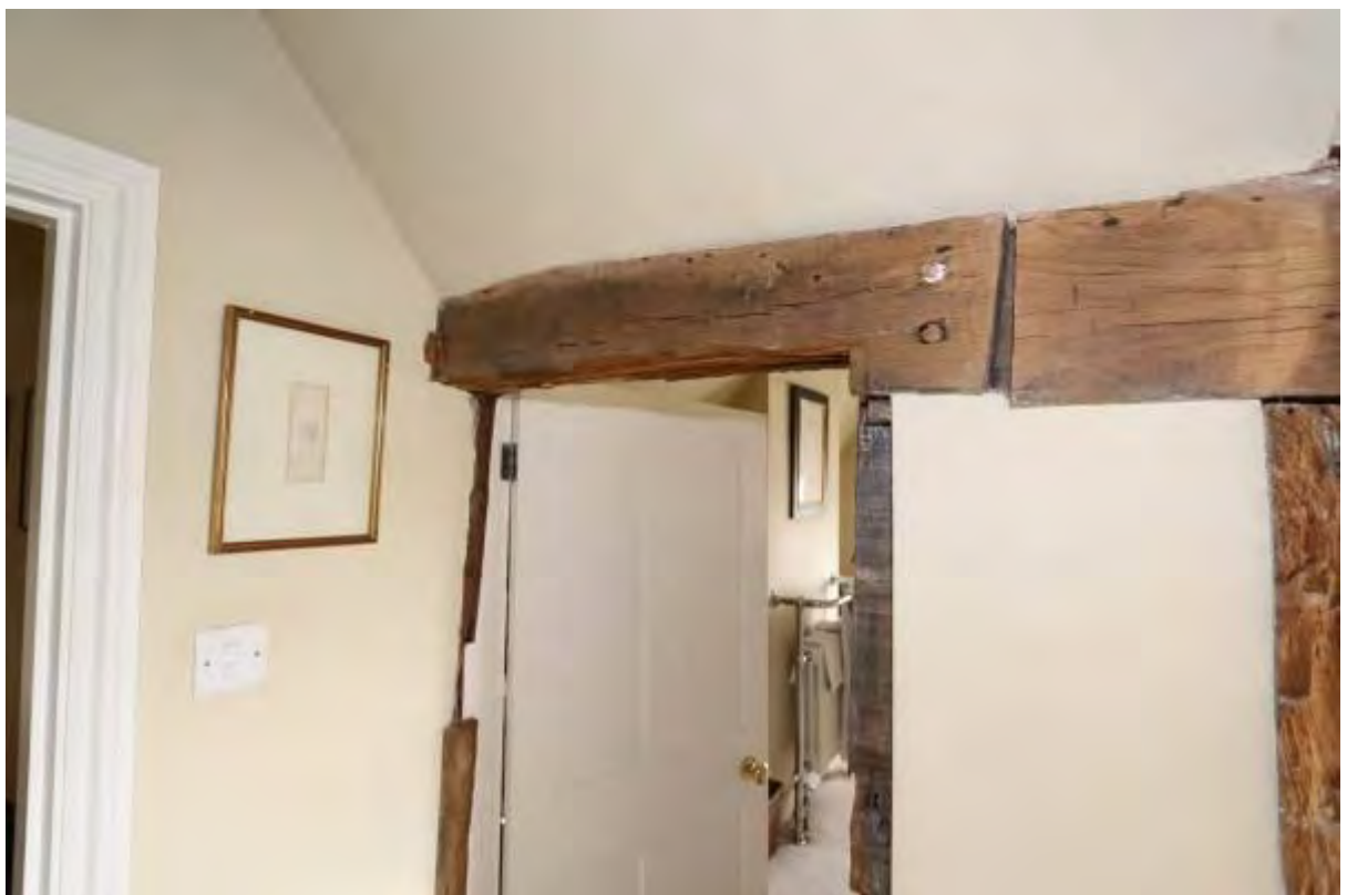
Plate 39 Cut away in wall plate for door opening (F4)
