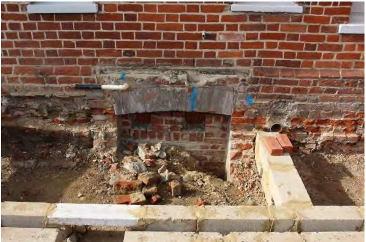
Plate 58 Blocked mid 19 th century window to basement
