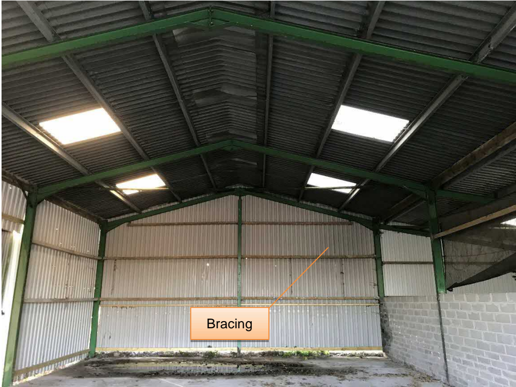
Photo 3: Roof Bracing
