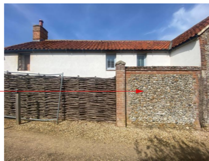
Existing brick and flint wall with coping stones.
