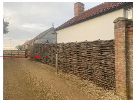
Woven Willow fence to be removed (Previously approved - PF/23/0339).
