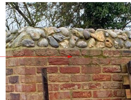
Proposed flint stone capping as commonly seen in Binham.
