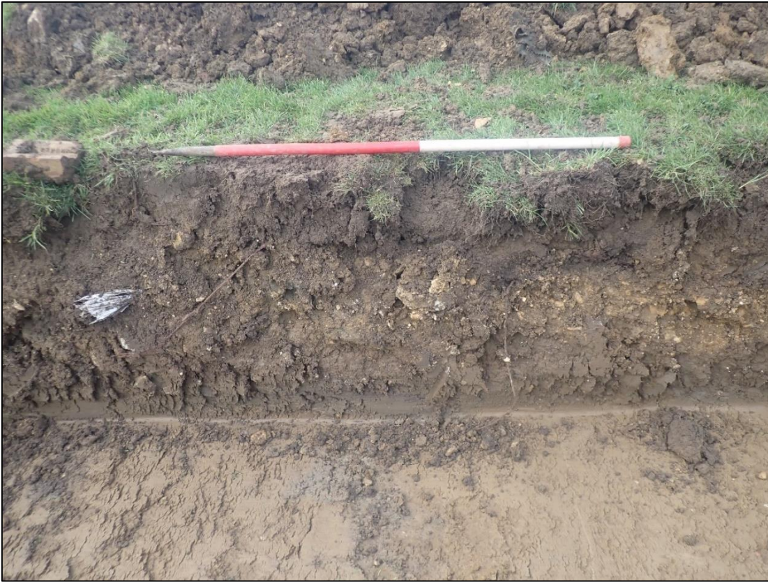
Trench 2: Baulk section from top to bottom: turf (20), make-up (21), make-up (22), subsoil (24), and undisturbed geology (23), looking south-west, 1m scale
