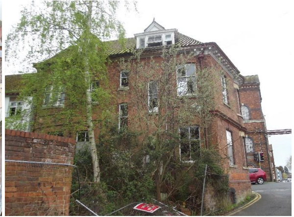
Northern and western elevations
