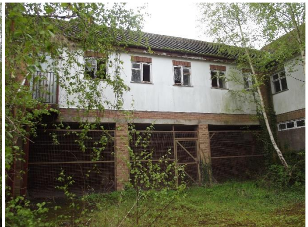
Western elevation eastern part
