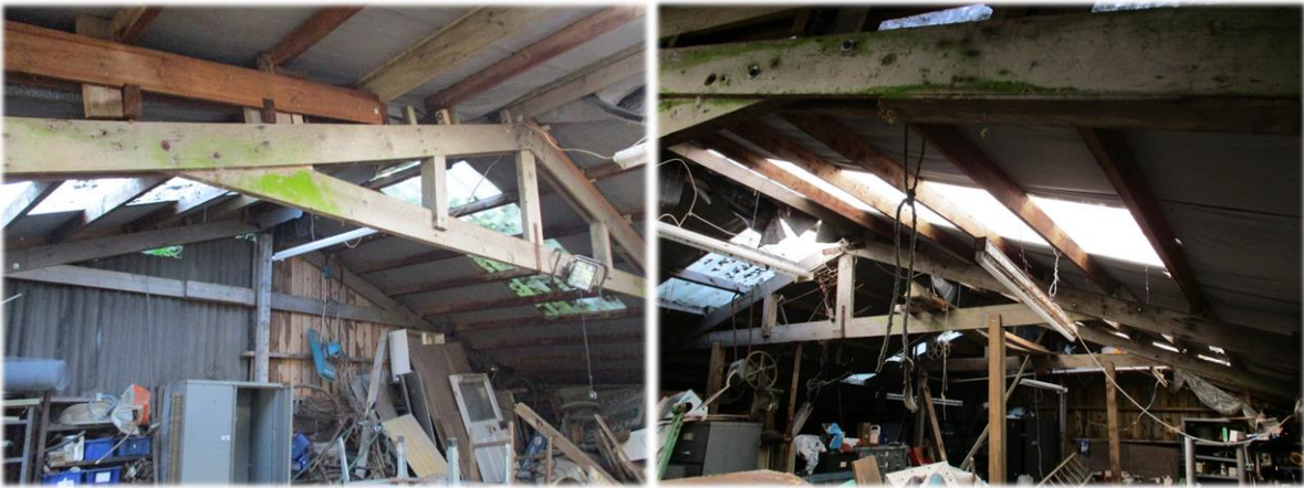
Storage barn interior
