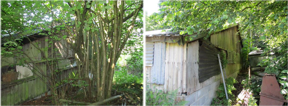
Storage barn northeast end (left) and southwest end (right)
