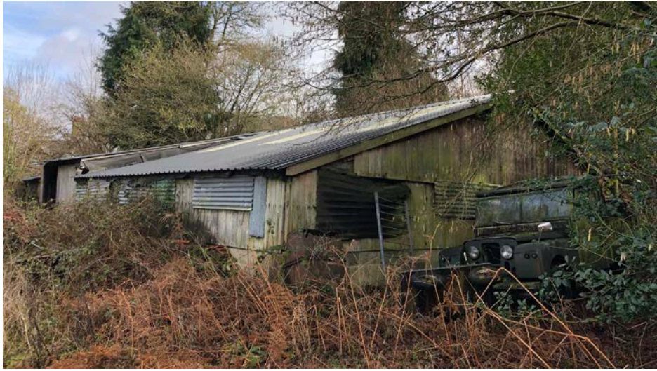
View of existing barn looking north east
