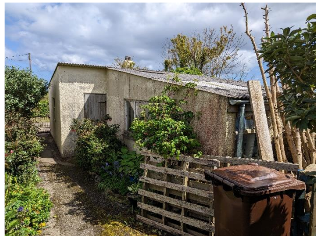
Photo 2. Showing the garage from the west
