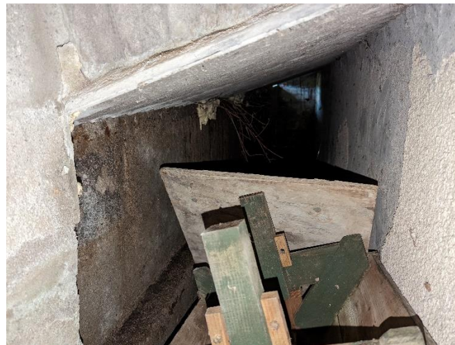
Photo 5. Showing the interior of the passage
