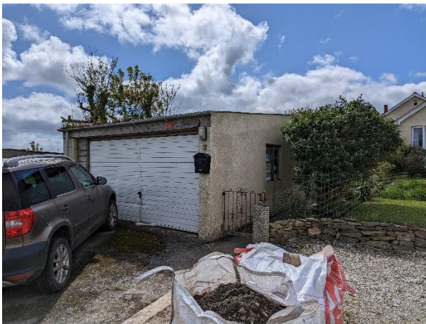
Photo 1. Showing the garage from the east
