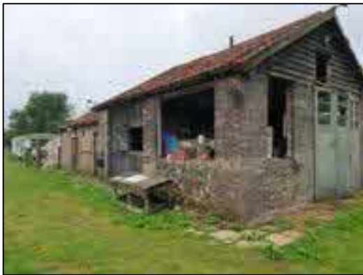
Figure 3 - Brick/stone barn, north-western area of eastern meadow
