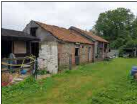
Figure 5 - Barn and stables viewed from south
