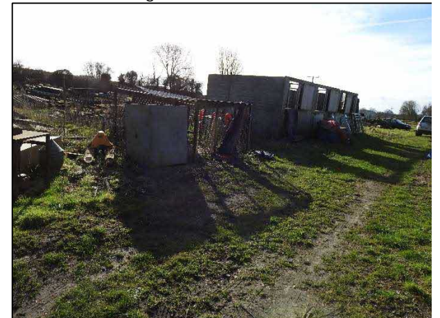
Derelict sheds to east of buildings
