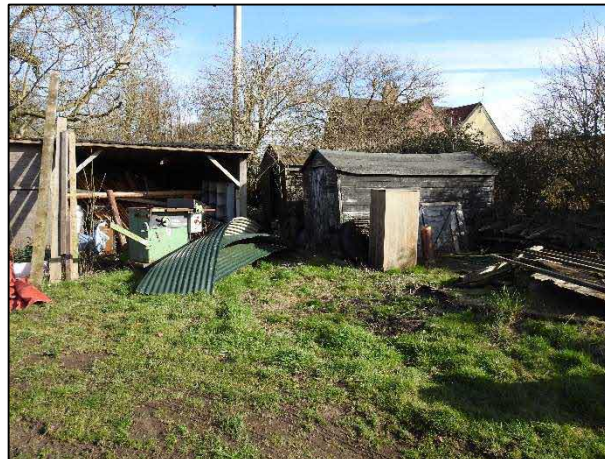
Derelict sheds of north of buildings
