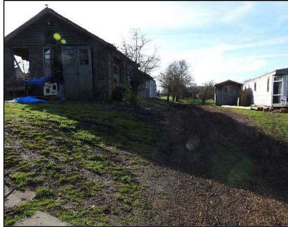
Access to caravans on west side of buildings
