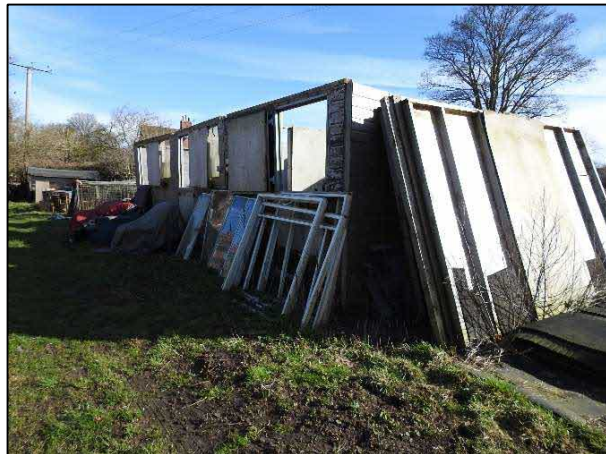
Stored materials to east of buildings
