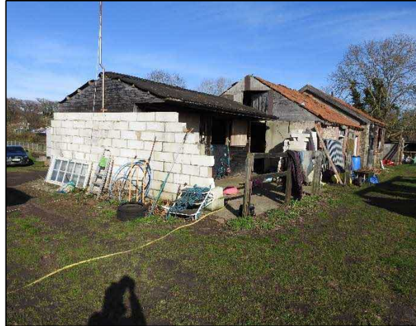
Barn and stables south end
