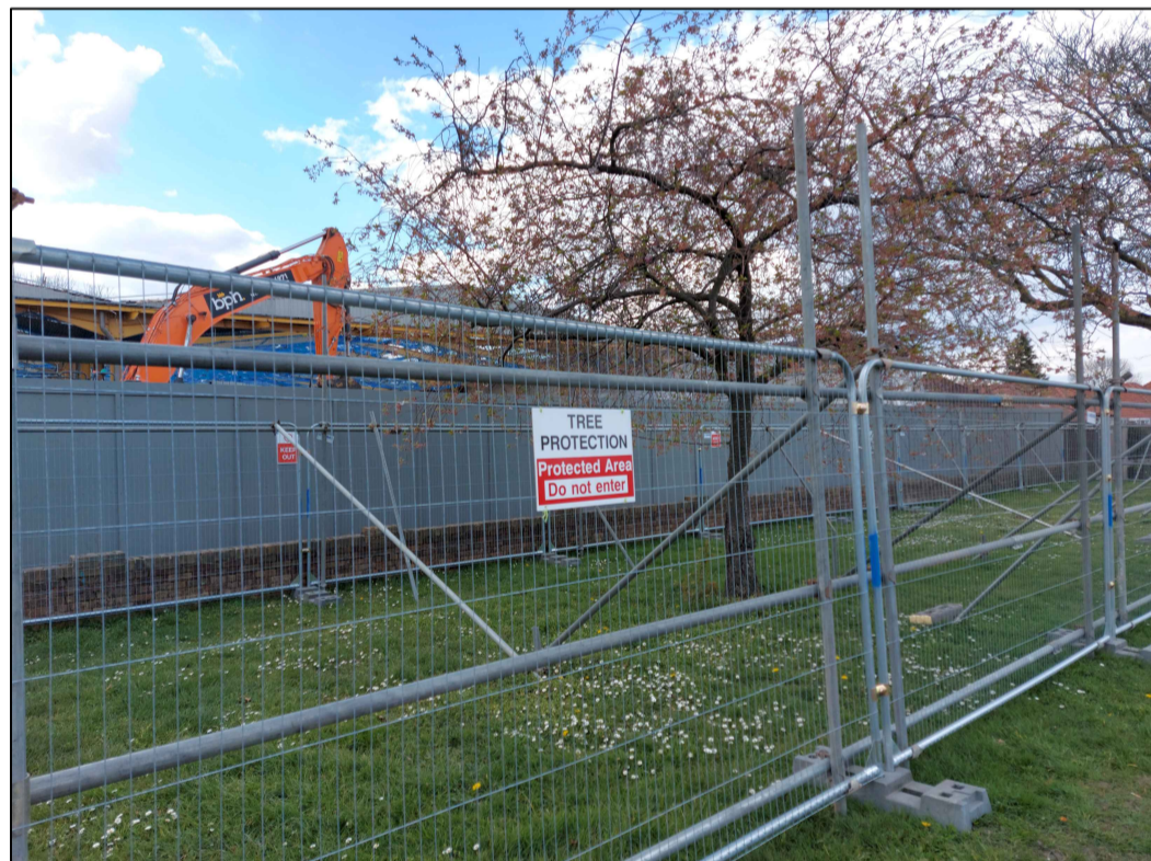
Security Fencing Example
