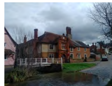
Principal West Elevation
