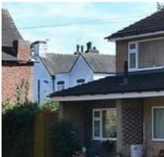
Image 10 View of Mavesyn Ridware House in context with Manor Croft
