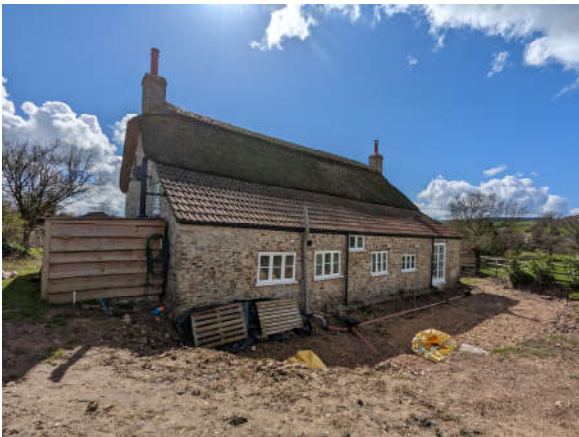
Rear elevation of Moxhayes
