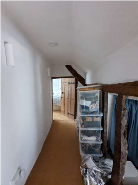
1 st floor hall showing timber frame
