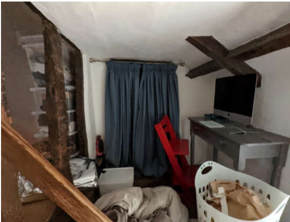
1 st floor hall at stairs
