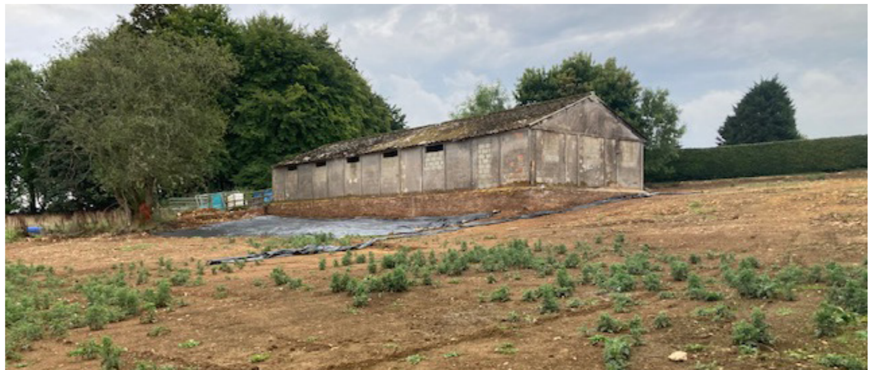
Existing 1930-40's concrete blockwork stable block
