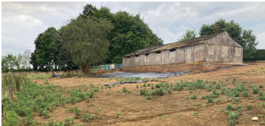
The Existing Stable Block
