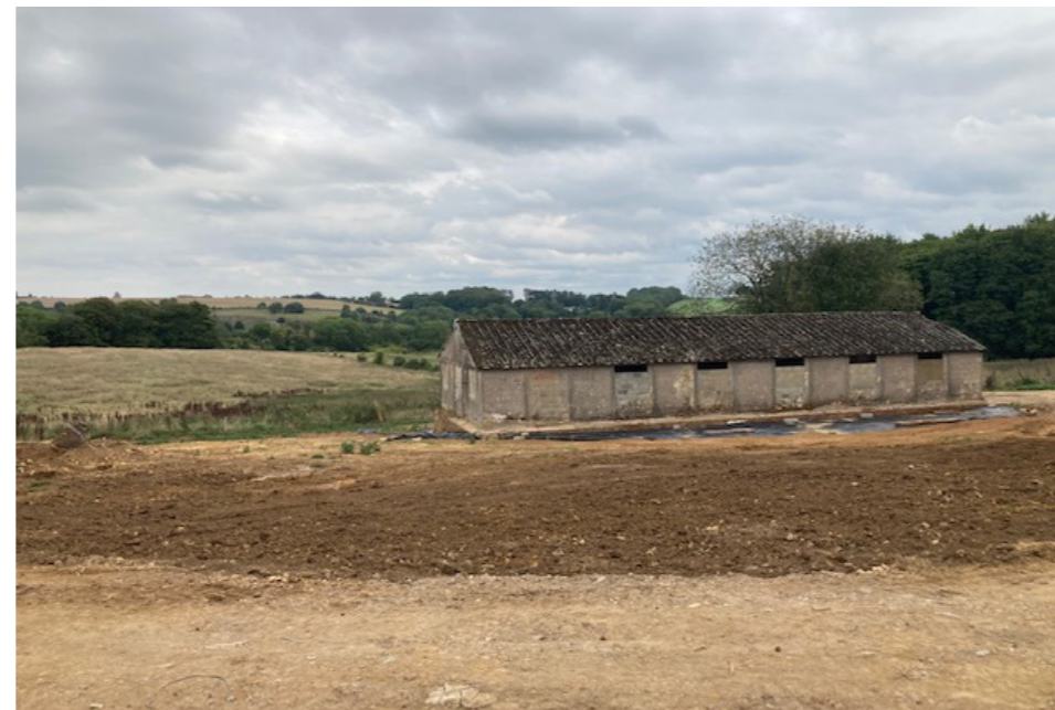
End of western elevation of the stable and view
