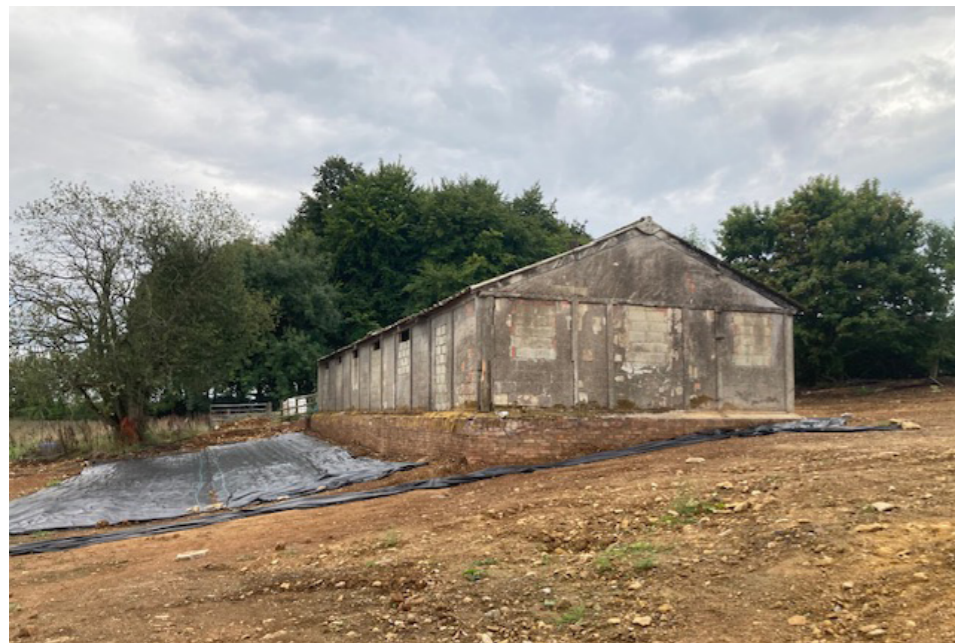
East and northern elevation of the stable
