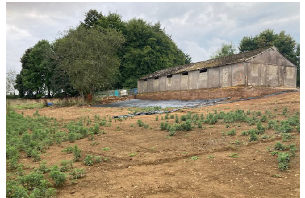
East and northern elevation of the stable
