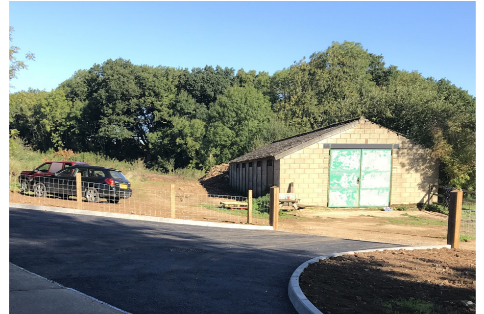
Western and southern elevations of the stable
