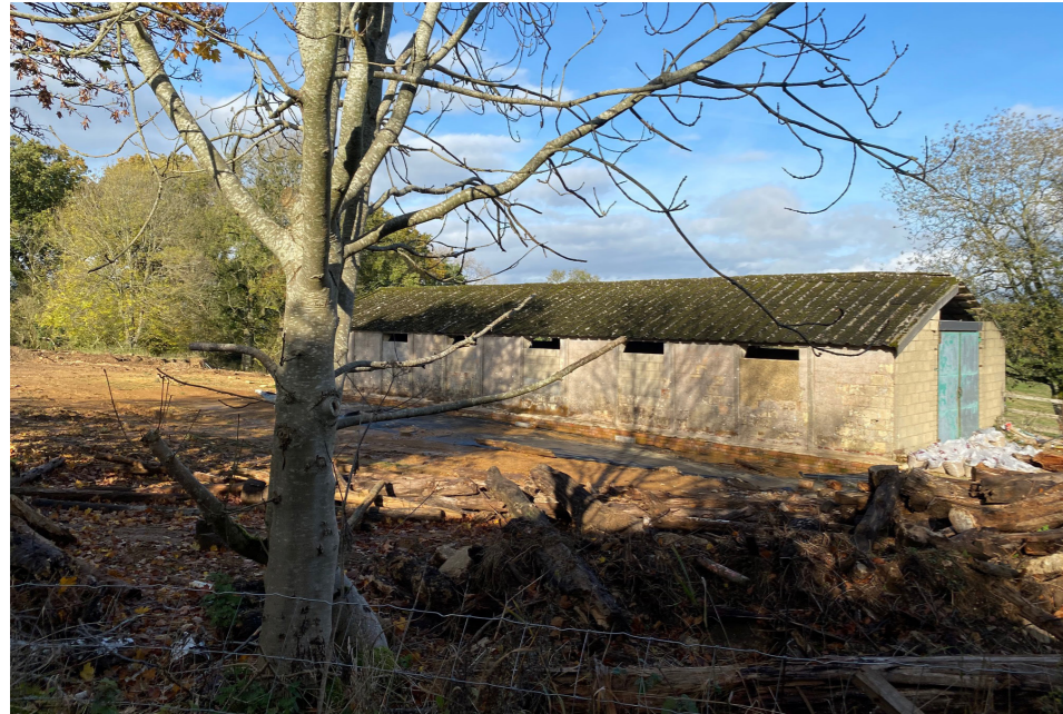
Western and southern elevations of the stable
