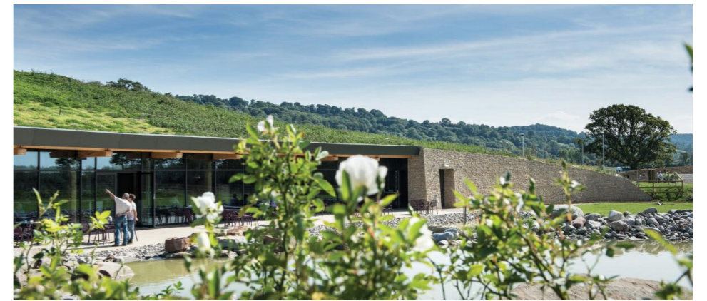
Gloucester M5 services, Glenn Howells Architects
