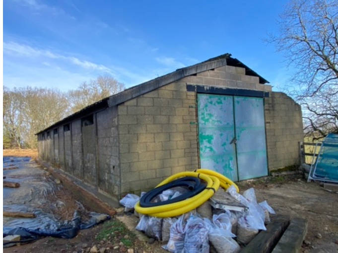
Photograph 6: View of the stable building from the south.
