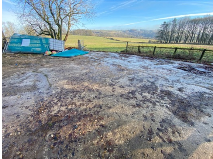
Photograph 2: Hard standing leading to the building in the southwest portion of the site.
