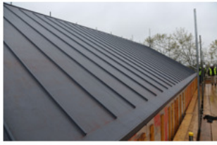
Standing Seam Single Ply Roof
