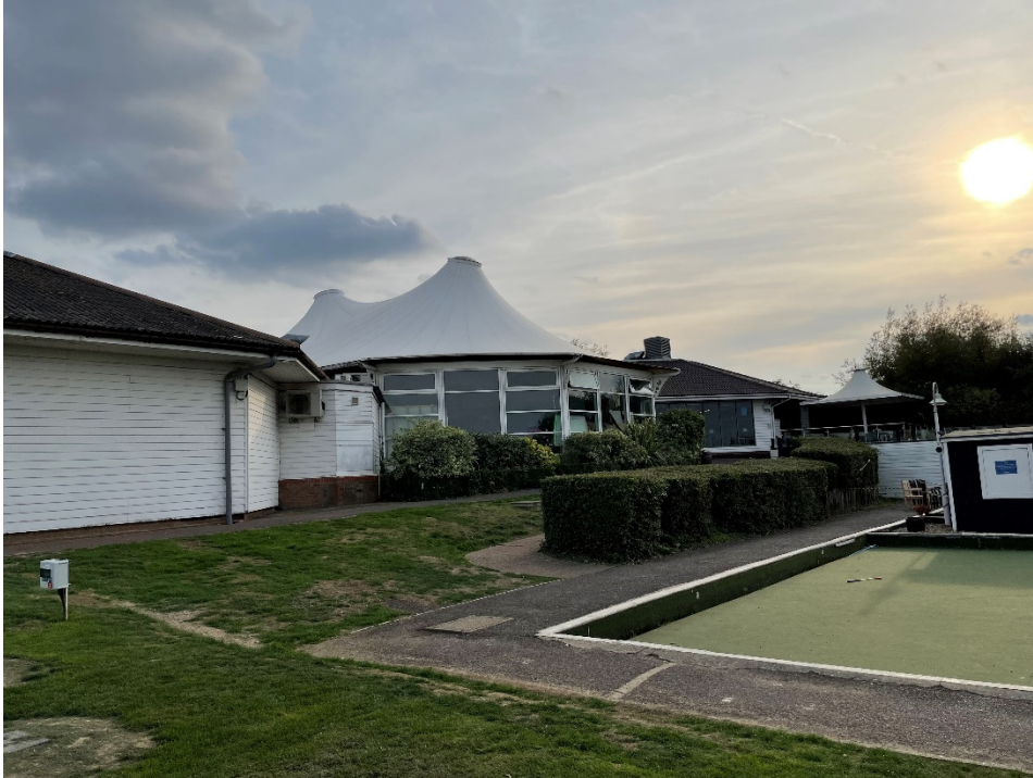
Existing building – Looking south west towards 'big top' between two blocks of main leisure building
