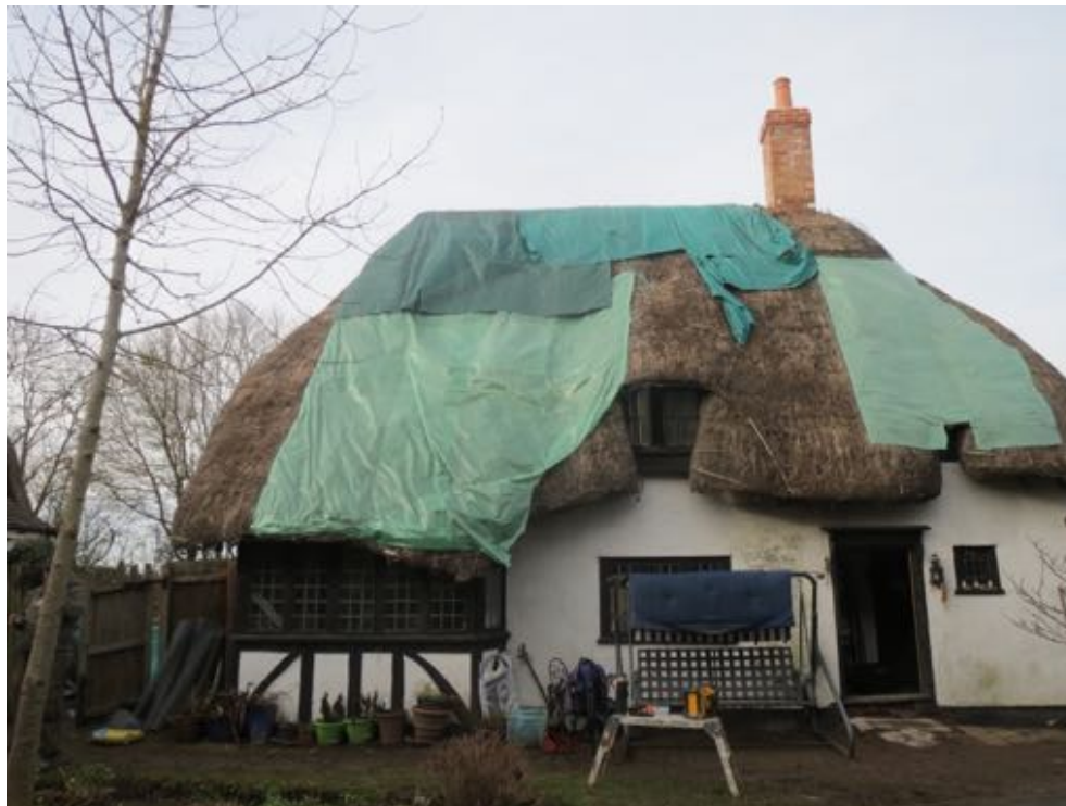
Elevation (rear) facing South-East
