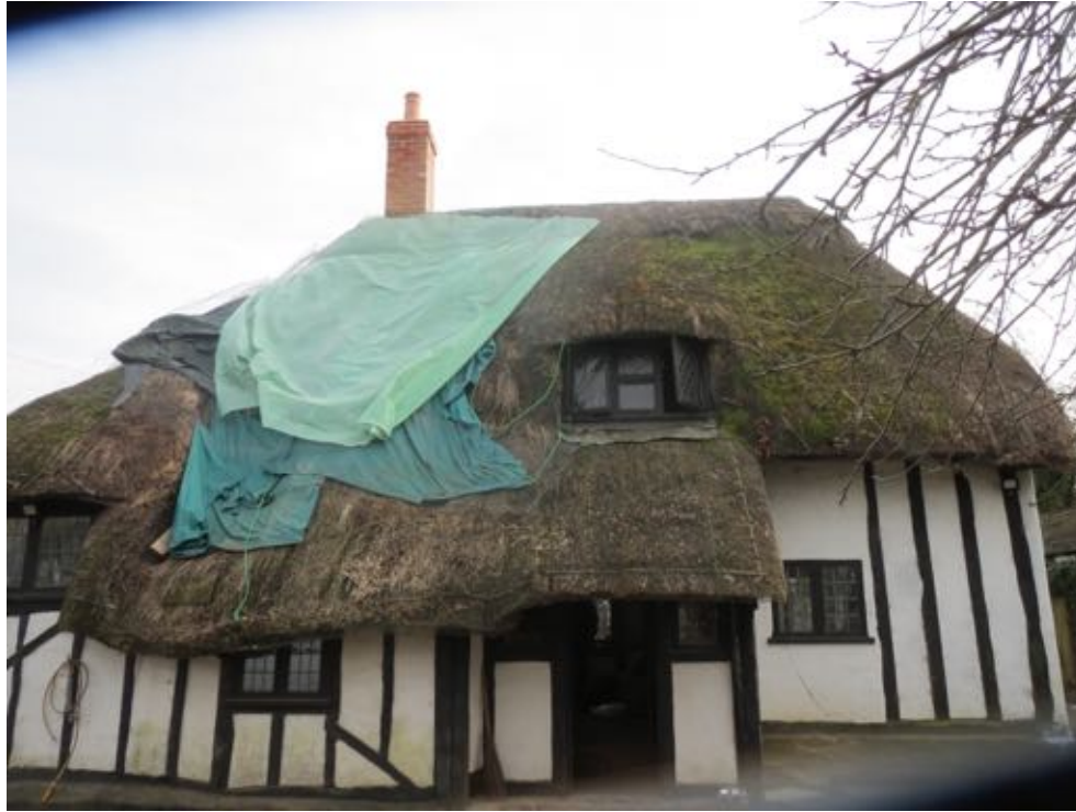
Elevation (front) facing North-West
