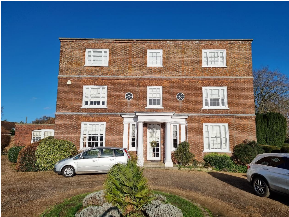
Fig.17: The south elevation of Langley Park House.
