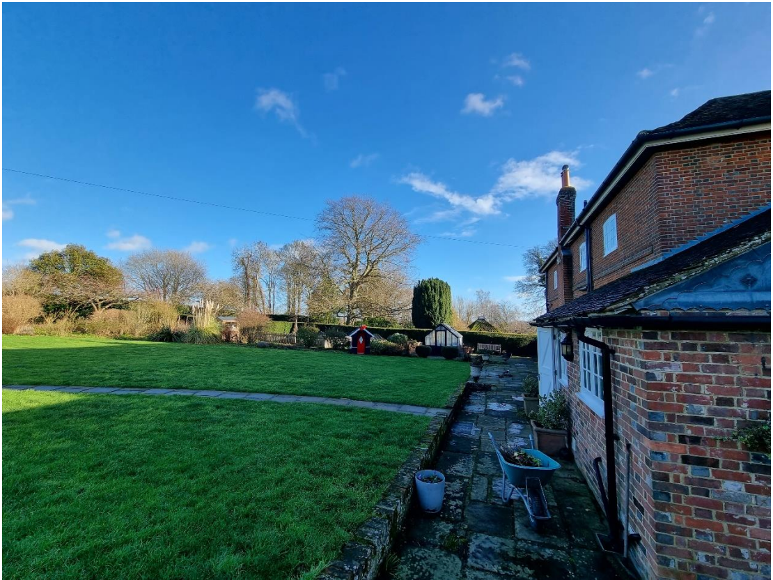
Fig.16: Looking in the direction of the site from the rear of Langley Park House. The topography and verdancy screens it from view.
