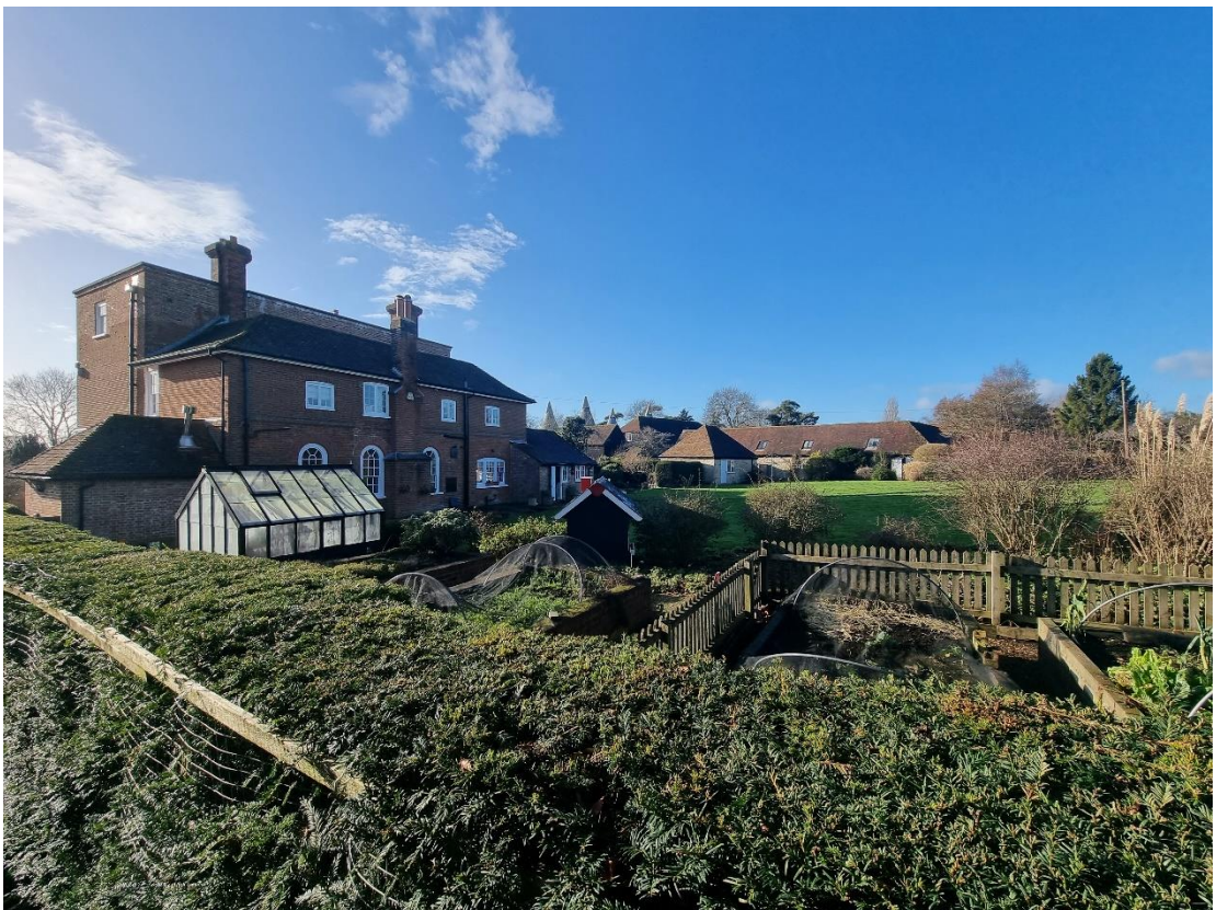
Fig.15: The rear and garden of Langley Park House, looking away from the site.
