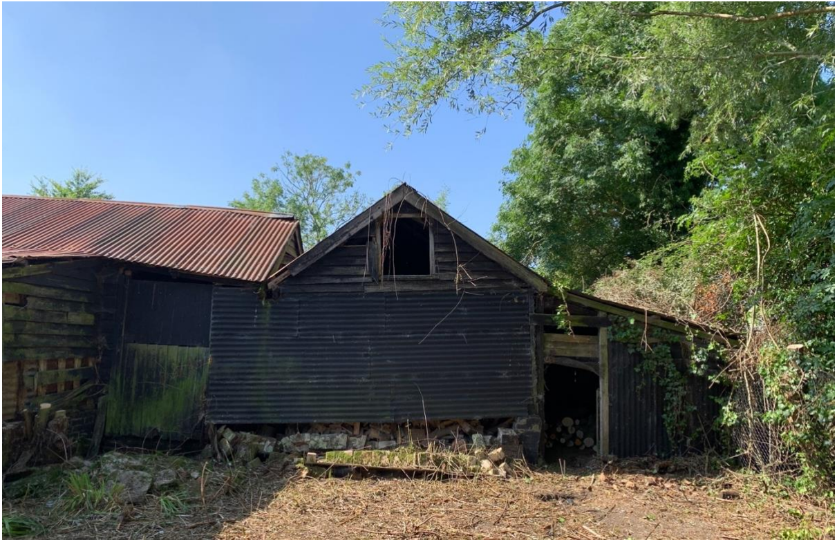
VIEW OF REAR OF OLD OUTBUILDING FOR DEMOLITION
