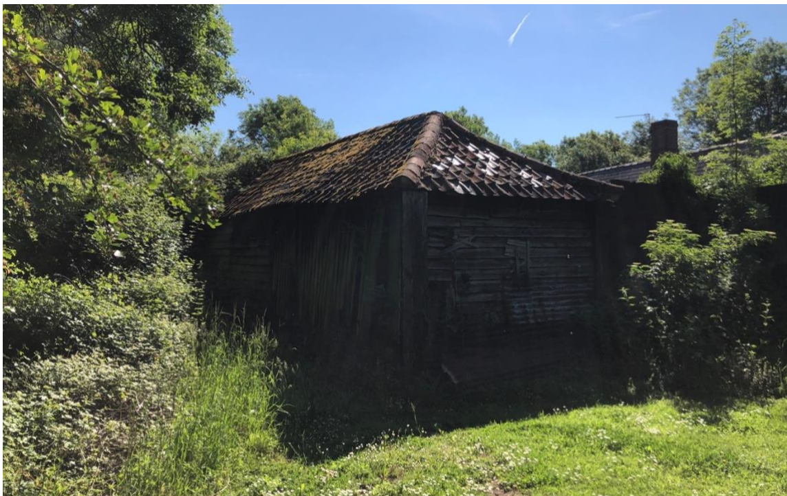
VIEW OF HIGHWAY FRONTING HIPPED ROOF END OF OUTBUILDING
