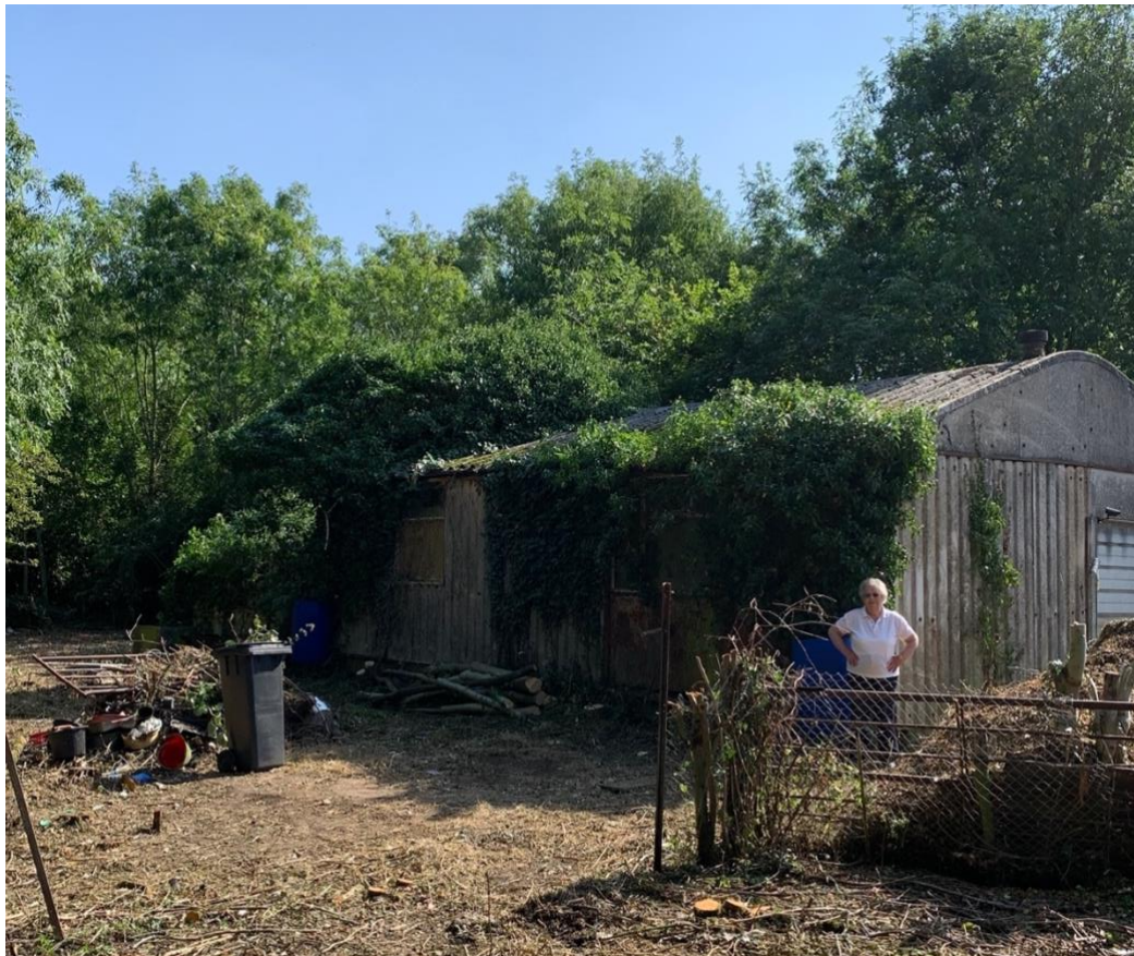
VIEW OF STEEL AND SHEET MATERIAL COVERED GARAGE/OUTBUILDING
