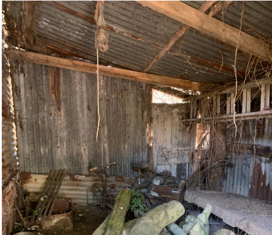
INTERNAL VIEW OF OUTSHOT
