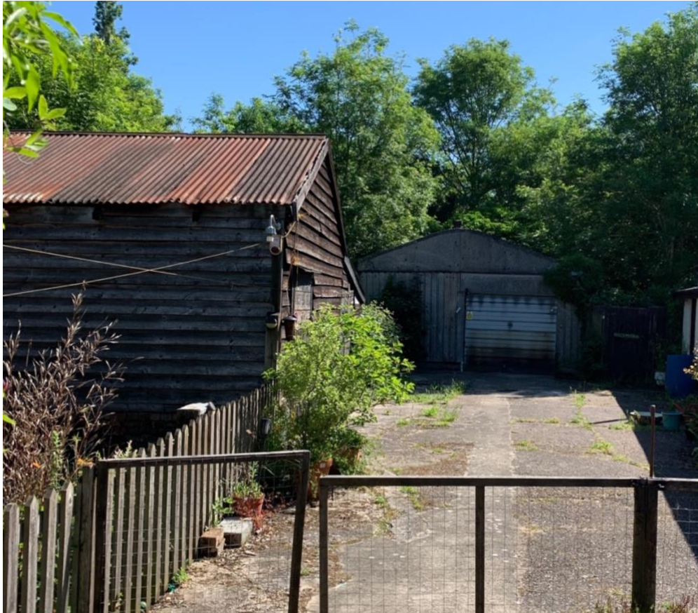
VIEW UP REAR COURTYARD/DRIVEWAY TO METAL CLAD BARN/GARAGE AT REAR
