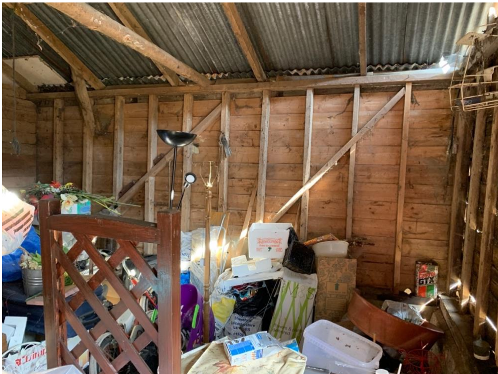
INTERNAL VIEW OF BARN
