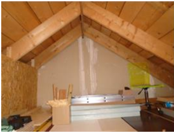
Figure 4 Interior of the loft (below).
