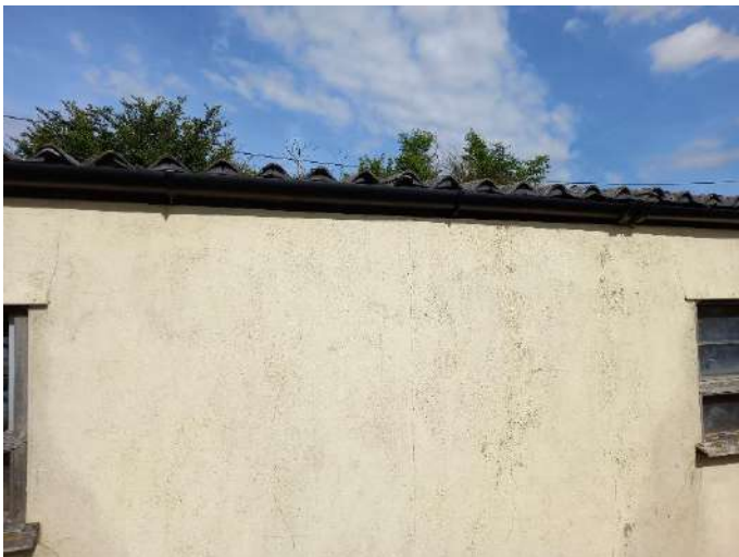
Figure 8: Possible ACM roofing material.
