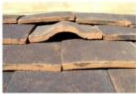
Example of bat access tile available from Tudor Clay Roof Tiles ( http://tudorrooftiles.co.uk/ )
