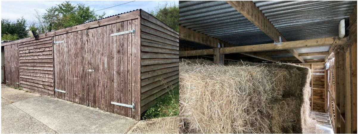
Fig 2 & 3. Hay store B1 to be demolished (left) and internal view of B1 (right)
