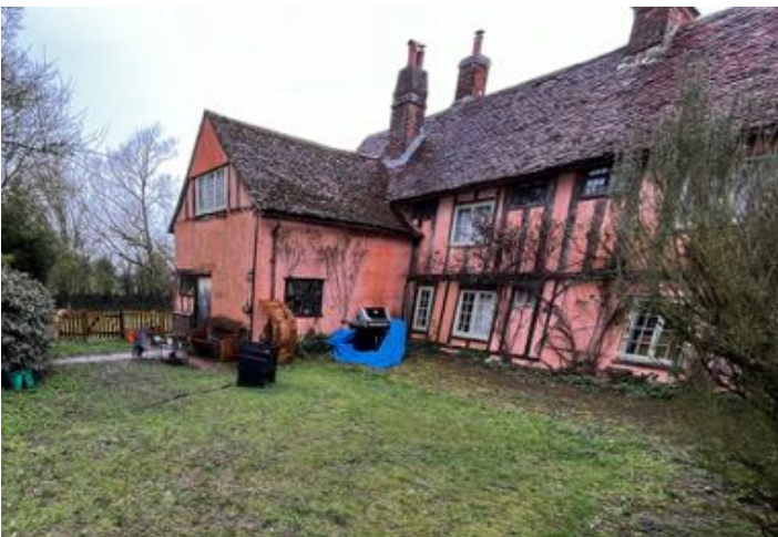
Outside photos of South Elevation of Dwelling
