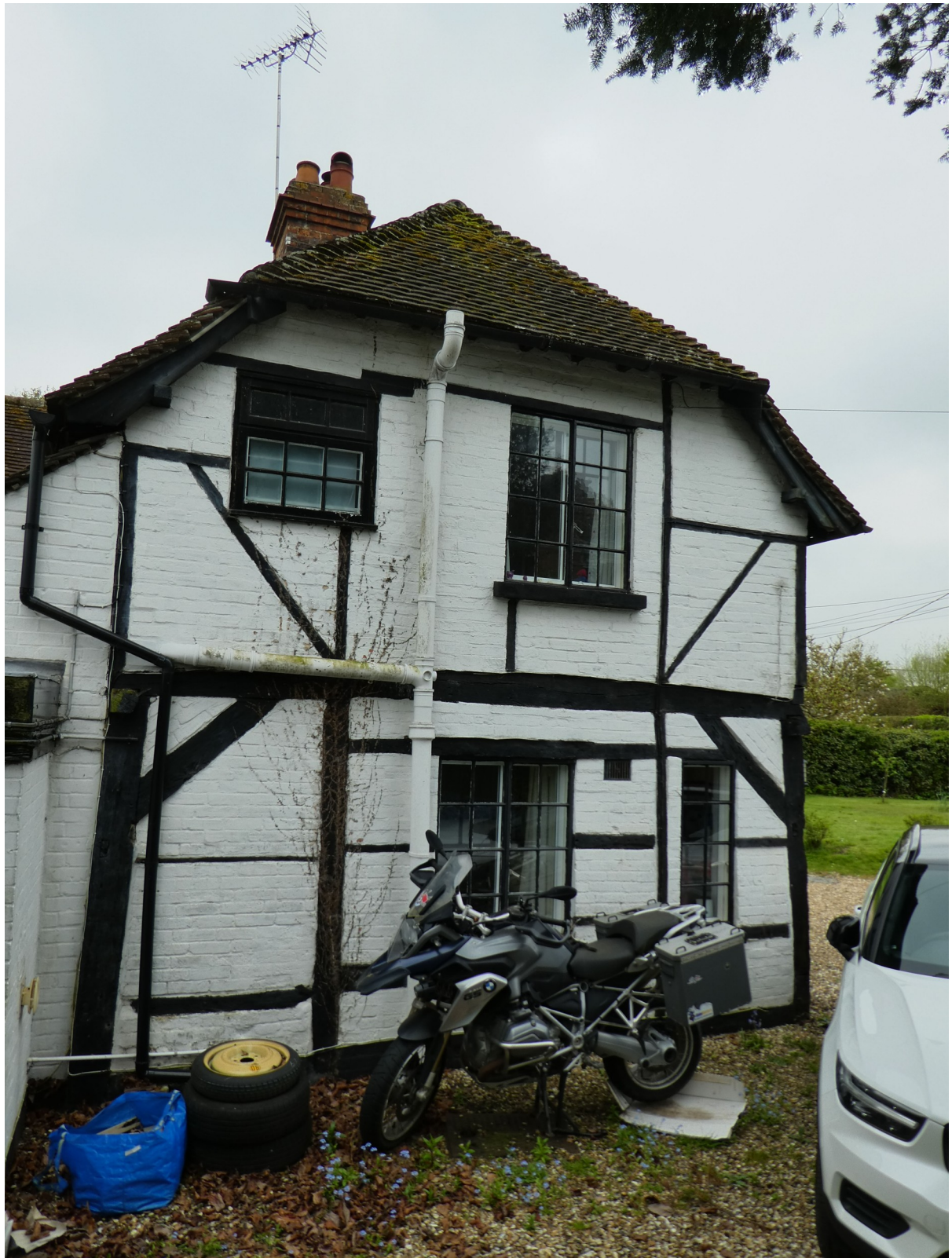
Photo 7 – Windows W14, W15, WF6 and WF7
