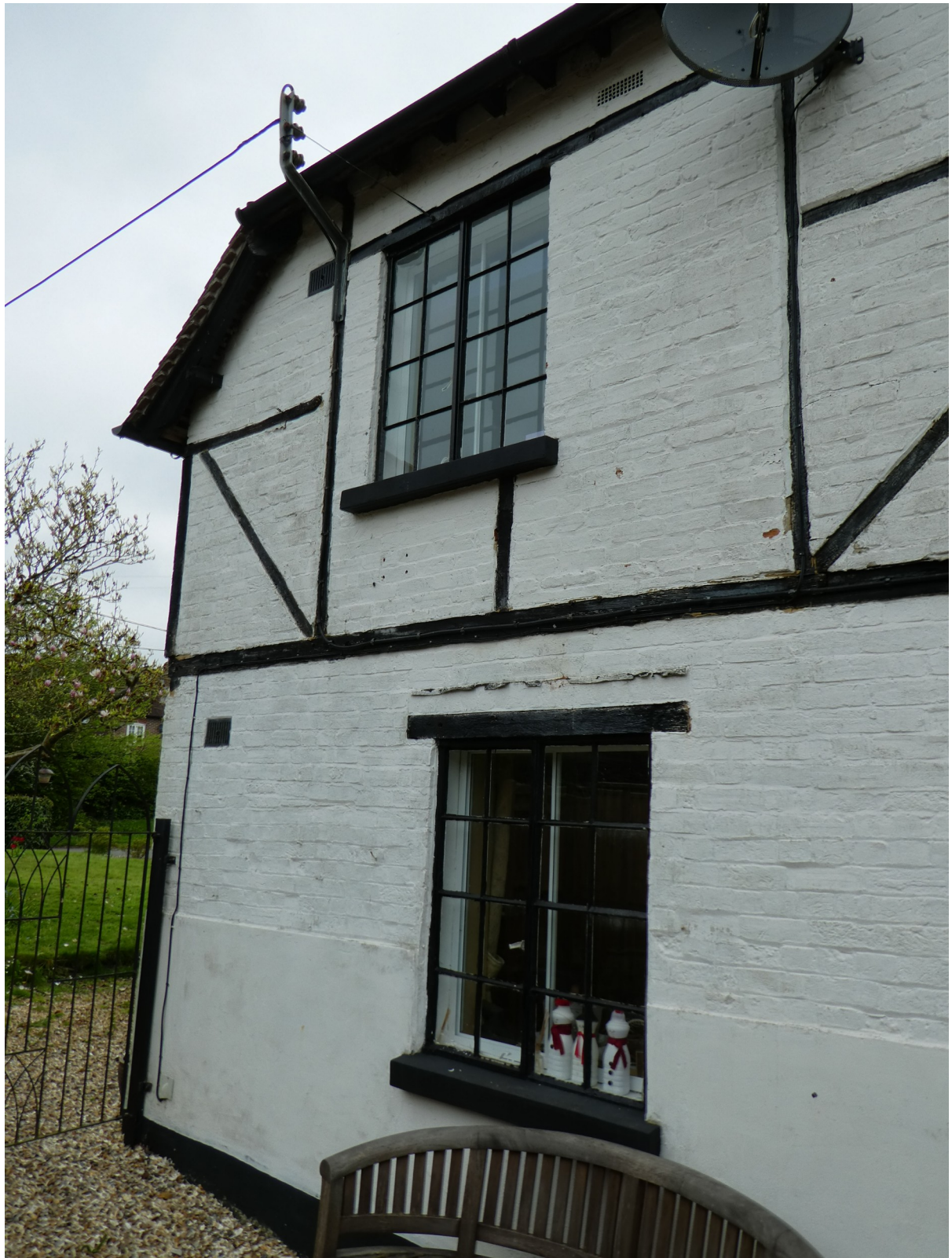
Photo 5 – Windows W3 and WF2
