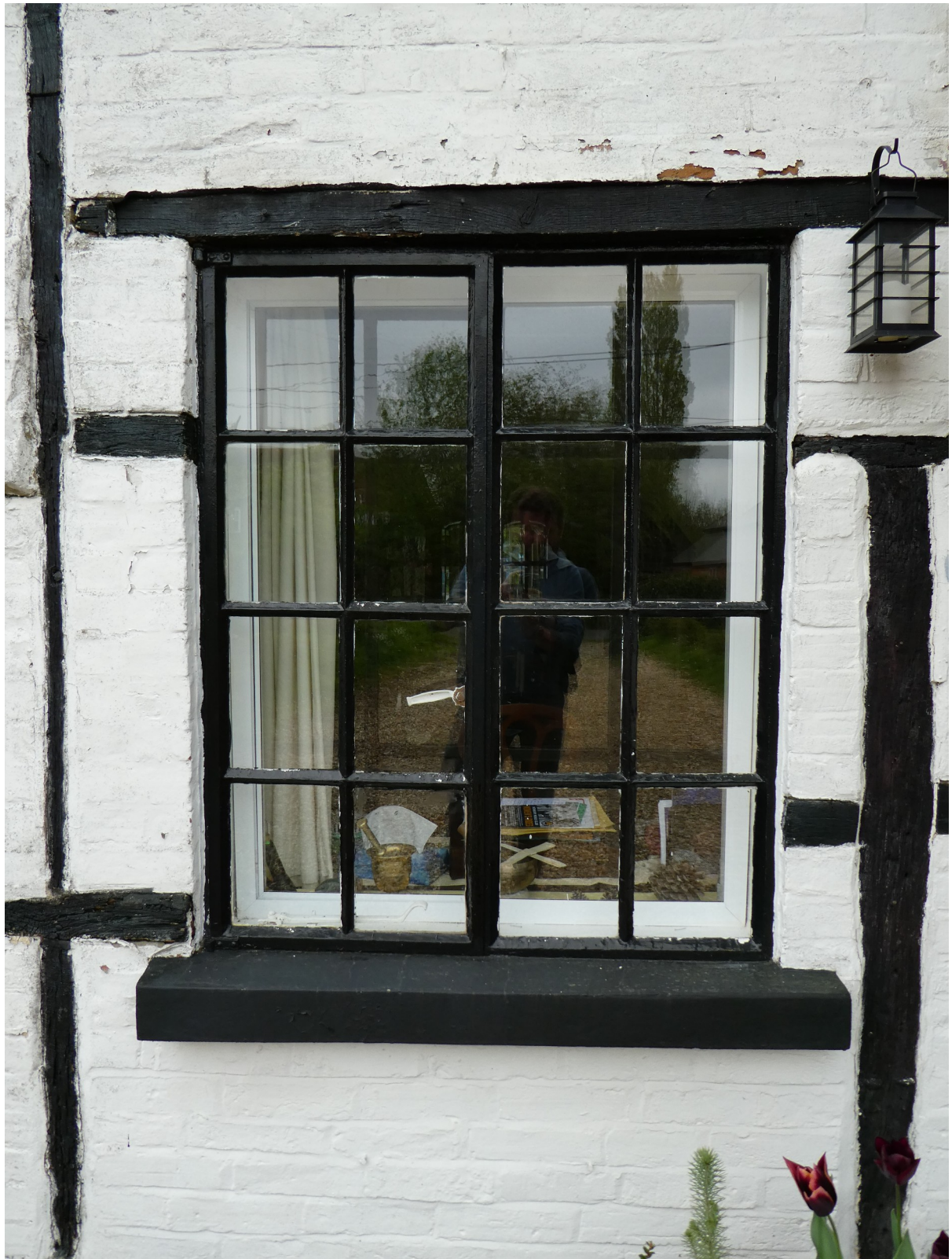
Photo 3 – Window W16 close up
