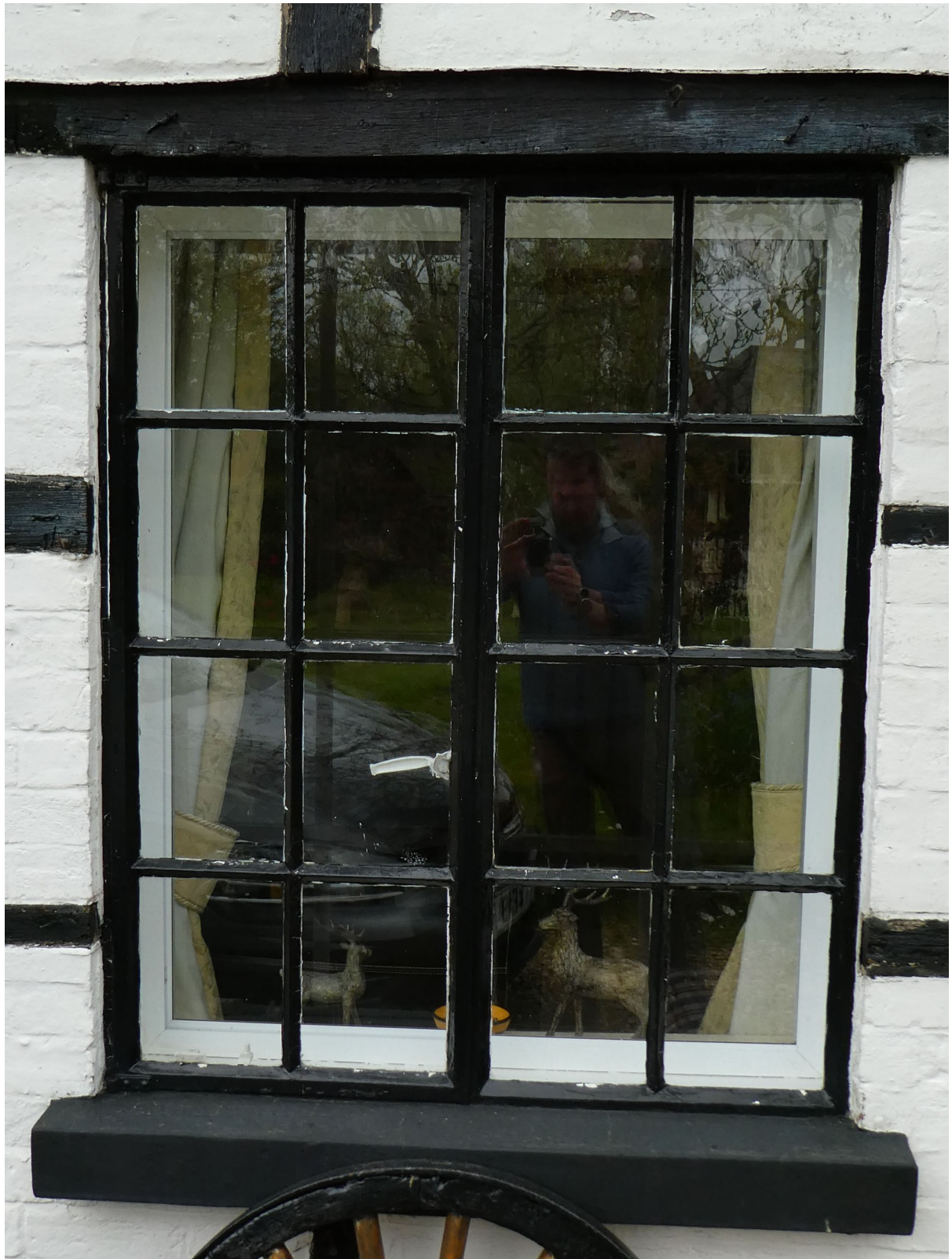
Photo 4 – Window W2 close up
