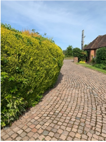
Figure 5 – Encroachment of hedge to courtyard
