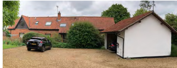
Fig 1.3: Image of the converted stables (red barn) and the garage
