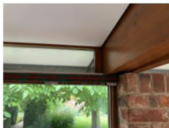
above view within hall of link block showing large glazing areas and exposed timbers of the roof construction top right the roof timbers continue through the elevation forming "cold-bridges" middle right the kitchen with louvred vents between the joist ends and distorted and decayed large opening lights below left to right details of shadow gap abutments of ceiling, roof timbers and recessed strip lights - forming draught penetrations of the construction. Single ply roofing with uv-degraded polycarbonate 'turret' rooflights
