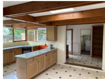
above view within hall of link block showing large glazing areas and exposed timbers of the roof construction top right the roof timbers continue through the elevation forming "cold-bridges" middle right the kitchen with louvred vents between the joist ends and distorted and decayed large opening lights below left to right details of shadow gap abutments of ceiling, roof timbers and recessed strip lights - forming draught penetrations of the construction. Single ply roofing with uv-degraded polycarbonate 'turret' rooflights
