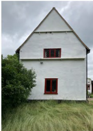
top views of the East elevation showing variation in window shapes and sizes within C20th flat cement render walls and new roof structure above left view of South elevation showing the leaded-light window and shedding boards retained/reinstated within the C20th reconstruction above right view of West elevation showing the leaded-light window are retained/reinstated within the C20th reconstruction
