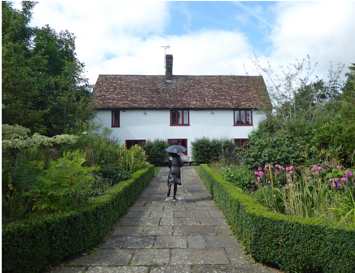
Fig 0.1: East Elevation of Hall Farmhouse from front garden - barn is to the left
