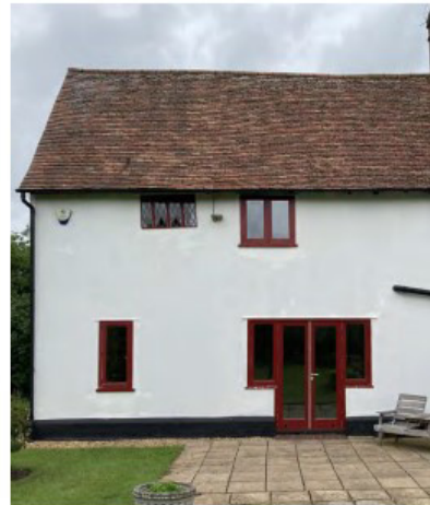
top views of the East elevation showing variation in window shapes and sizes within C20th flat cement render walls and new roof structure above left view of South elevation showing the leaded-light window and shedding boards retained/reinstated within the C20th reconstruction above right view of West elevation showing the leaded-light window are retained/reinstated within the C20th reconstruction
