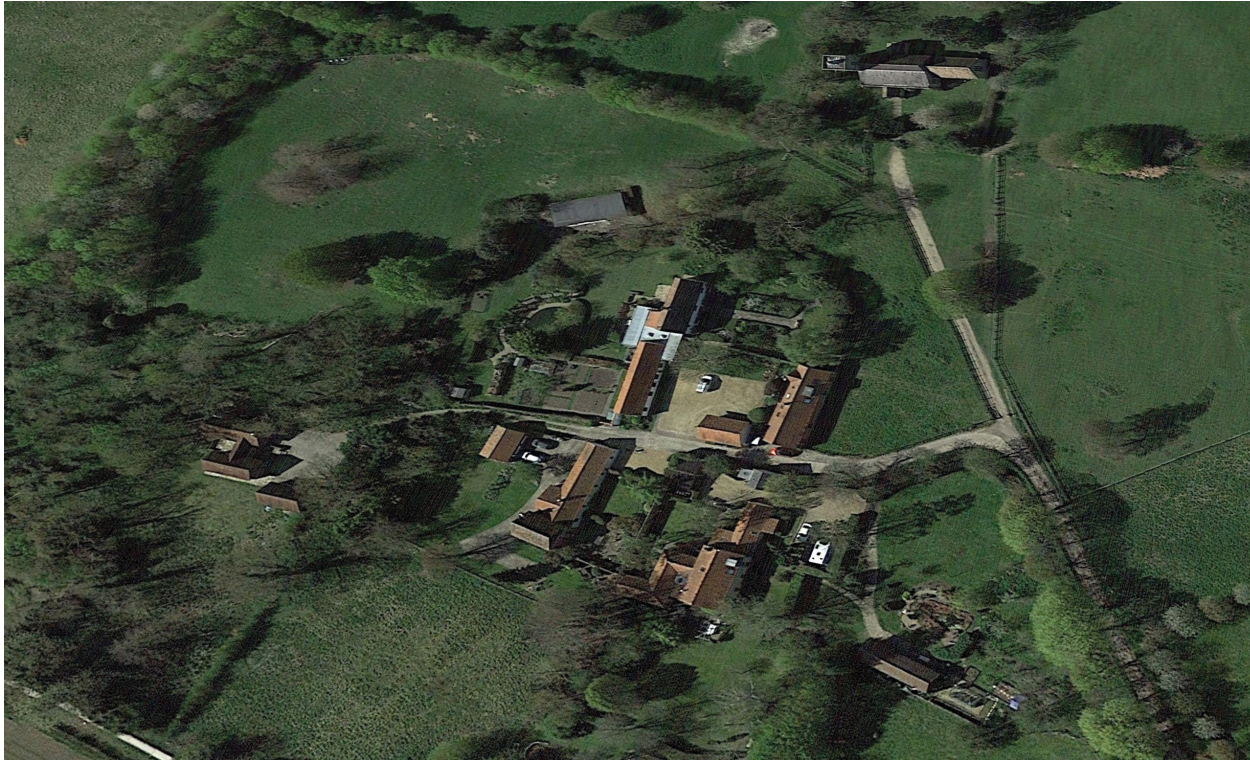
Fig 0.2: Aerial view of Hall farmhouse and wider context from SE google earth
