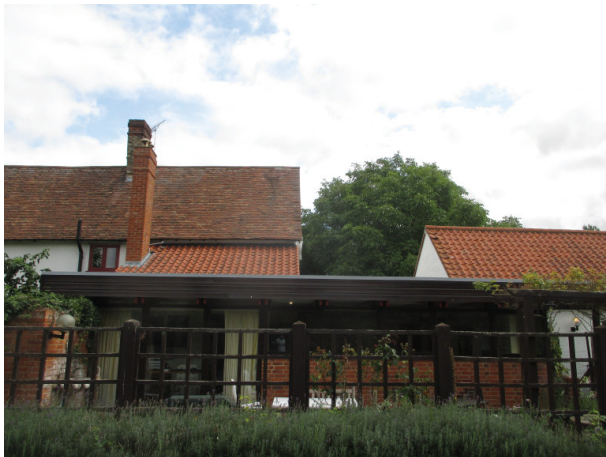
Fig 2.1 View showing separation of the farmhouse and the barn with the flat roof link from the private garden.
