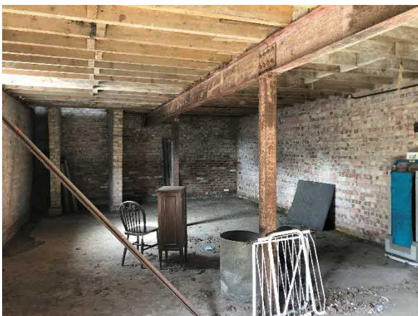
Photo 13: Internal view of B6, ground floor
