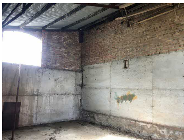
Photo 18: Internal view of B8
