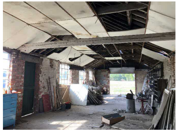
Photo 6: Internal view of B3
