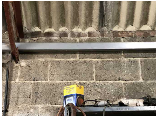
Photo 10: Internal view of B5 showing filled gaps around eaves
