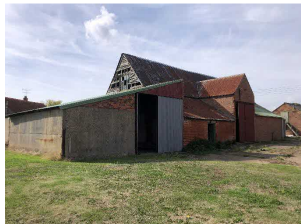
Photo 12: North eastern facades of B6, with adjoining to the east
