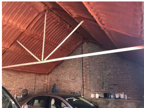
Photo 16: Internal view of B7, showing foam line roof
