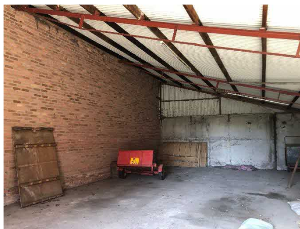
Photo 2: Internal view of B1
