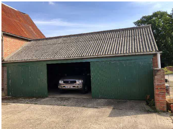
Photo 15: Western façade of B7, with B6 to north
