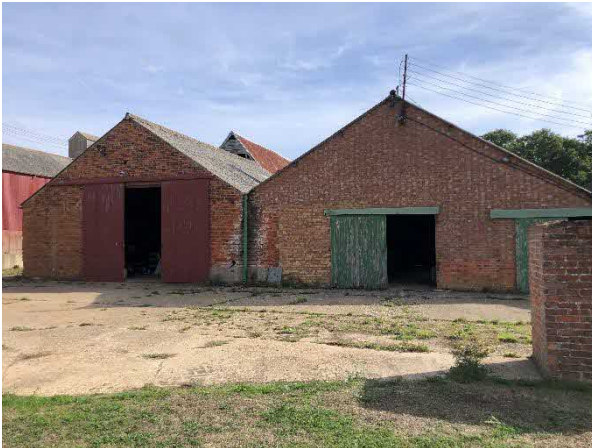
Photo 9: Western façade of B5
