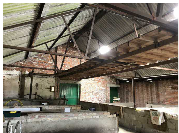
Photo 8: Internal view of B4
