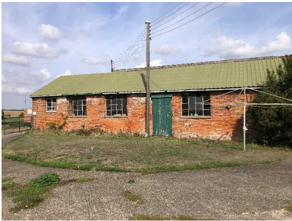
Photo 5: Southern facade of B3
