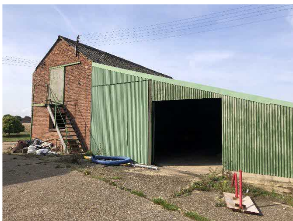
Photo 1: Eastern facade of B1, adjoining B2
