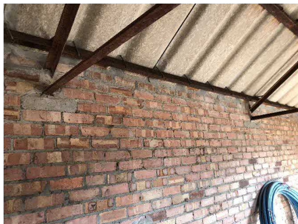
Photo 4: Internal view of B2, upper floor, showing cemented eaves
